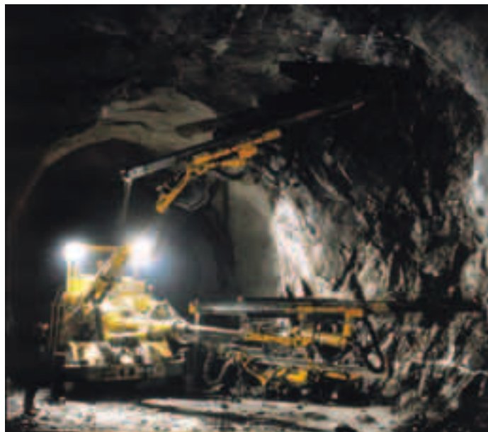
Tunneldrivning under mark.
