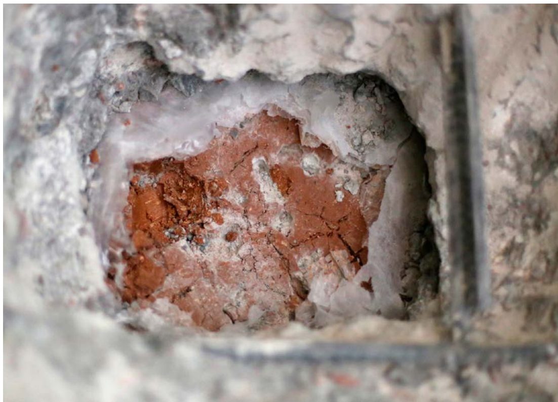
Figure 2-14. The silo bentonite as it looks in 2014. Picture is taken through a hole in the temporary lid.
