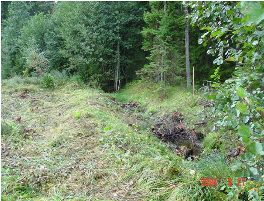
Figure 4-1. Cleaning of vegetation for installation of brook discharge gauging station PFM002667.
