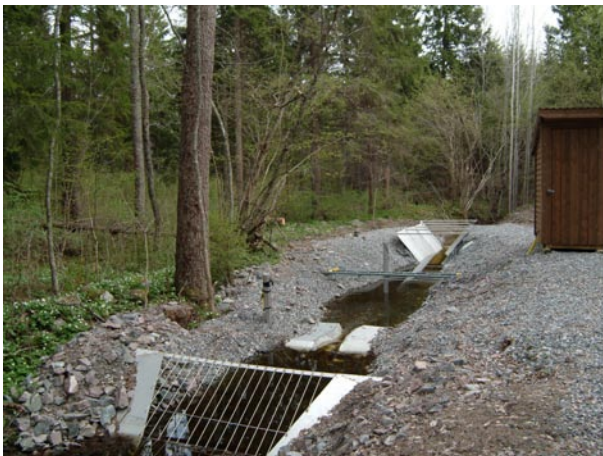
Figure A1-3. Top: After cleaning of vegetation in Sep. 2004. Middle: After excavation and refilling with crushed stone and gravel, Sep. 2004. Bottom: After installation in May 2005.
