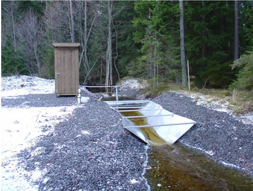
Figure 4-3. Discharge station PFM002667 with the large flume in the foreground, the small flume upstream in the background and the service module with the LPG burner to the left. The tube in the middle of the brook between the flumes is screened and used for installation of devices for measurement of electrical conductivity and temperature.
