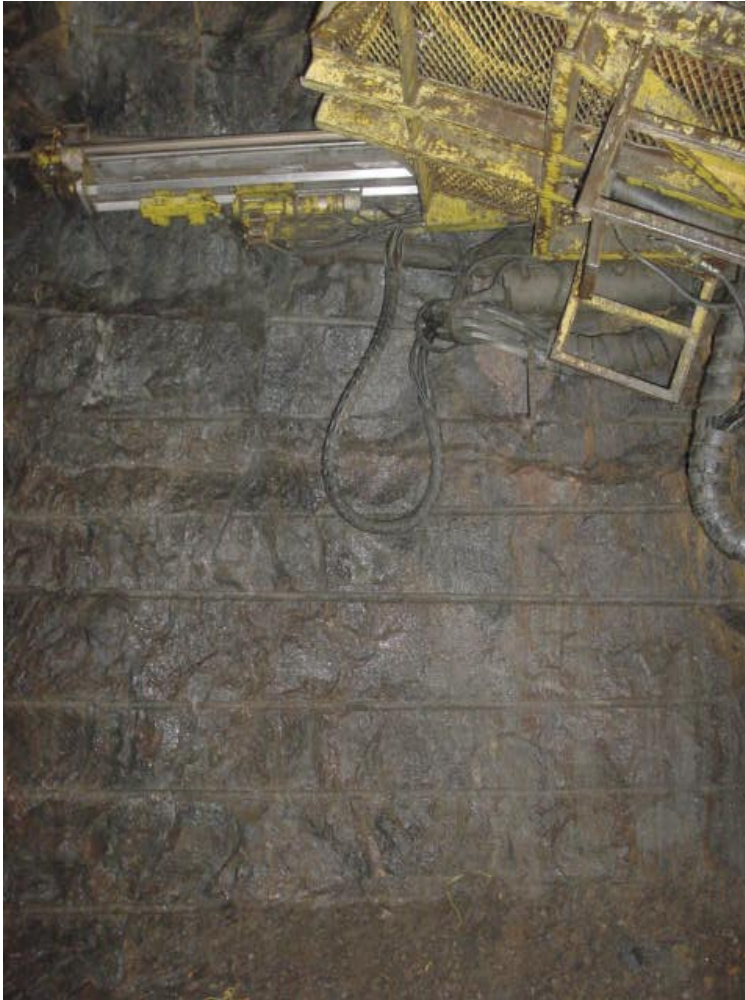
Figure 6-20. Half casts in the right hand wall of round 2.
