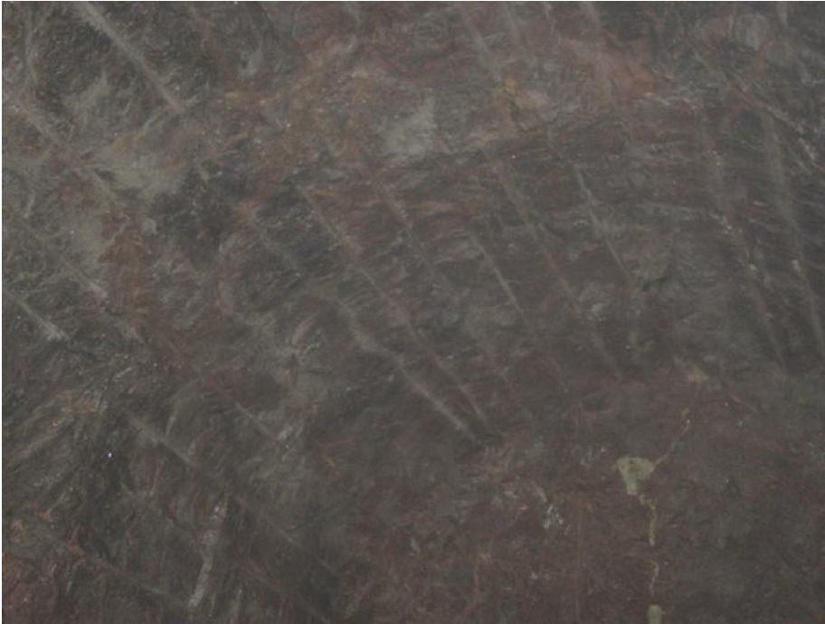
Figure 6-21. Half casts in the roof of round 3.
