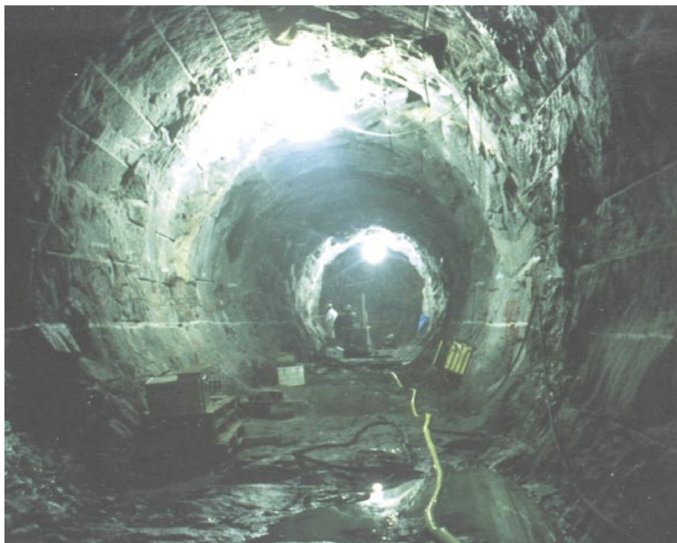
Figure 6-9. The circular shaped Zedex tunnel has a diameter of 5.0 m.
