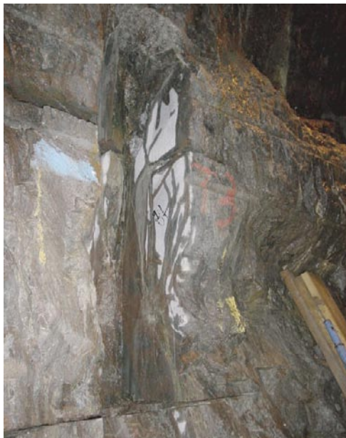
Figure 7-6. Right slot wall.
