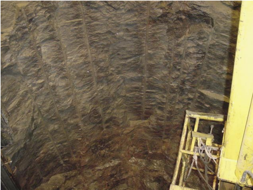
Figure 6-19. Round 2. Half casts in the roof. Notice spacing variation.
