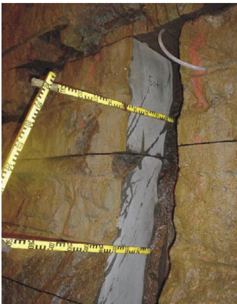
Figure 7-18. Cracks from the left slot wall.
