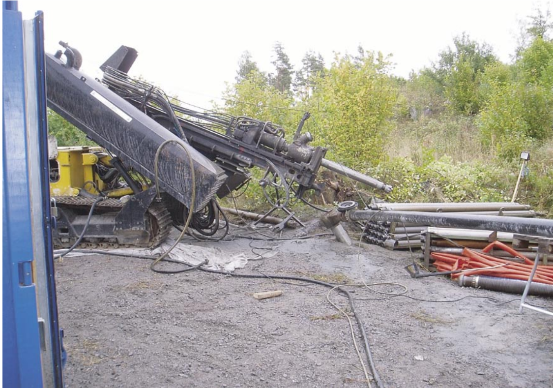
Figure 4-2. Drilling equipment at the site for HLX27.
