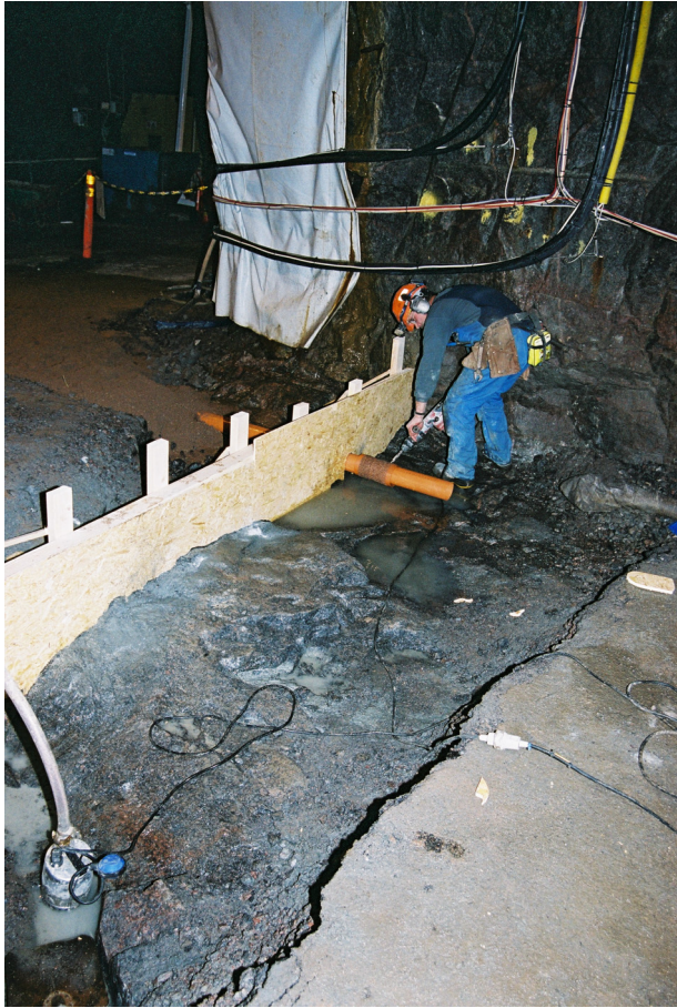
Figure 5-5 The concrete weir MG0004G during construction
