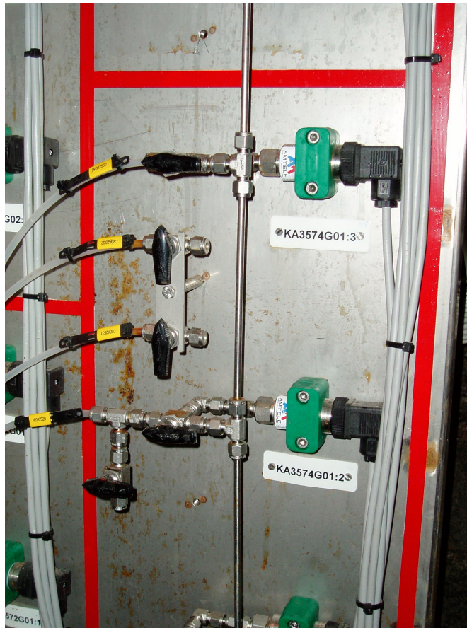
Figure 6-3 Pressure transducers connections
