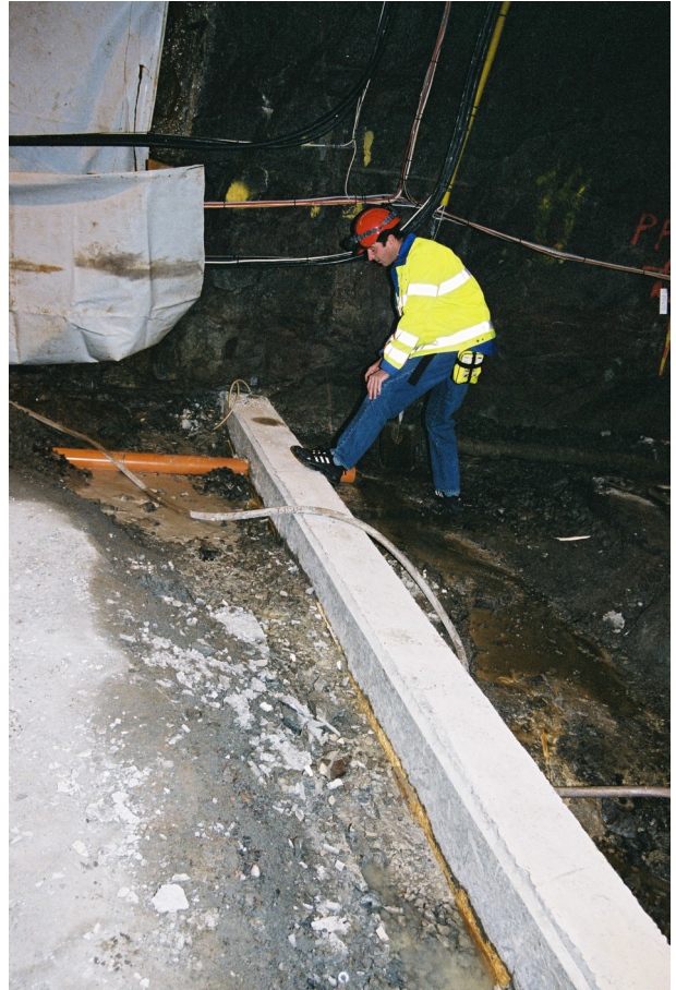
Figure 5-5 The concrete weir MG0004G during construction
