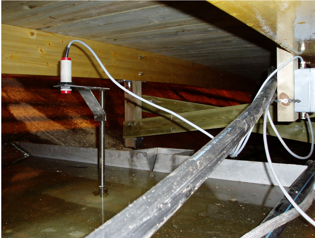
Figure 5-4 One of the three weirs downstream of plug 2 with the ultrasonic transmitter visible
