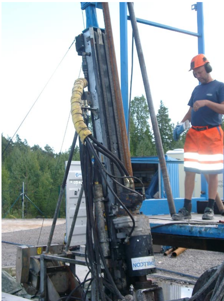
Figure 3-1. The Onram 1000 core drilling machine in operation on drillhole KFM01B.
