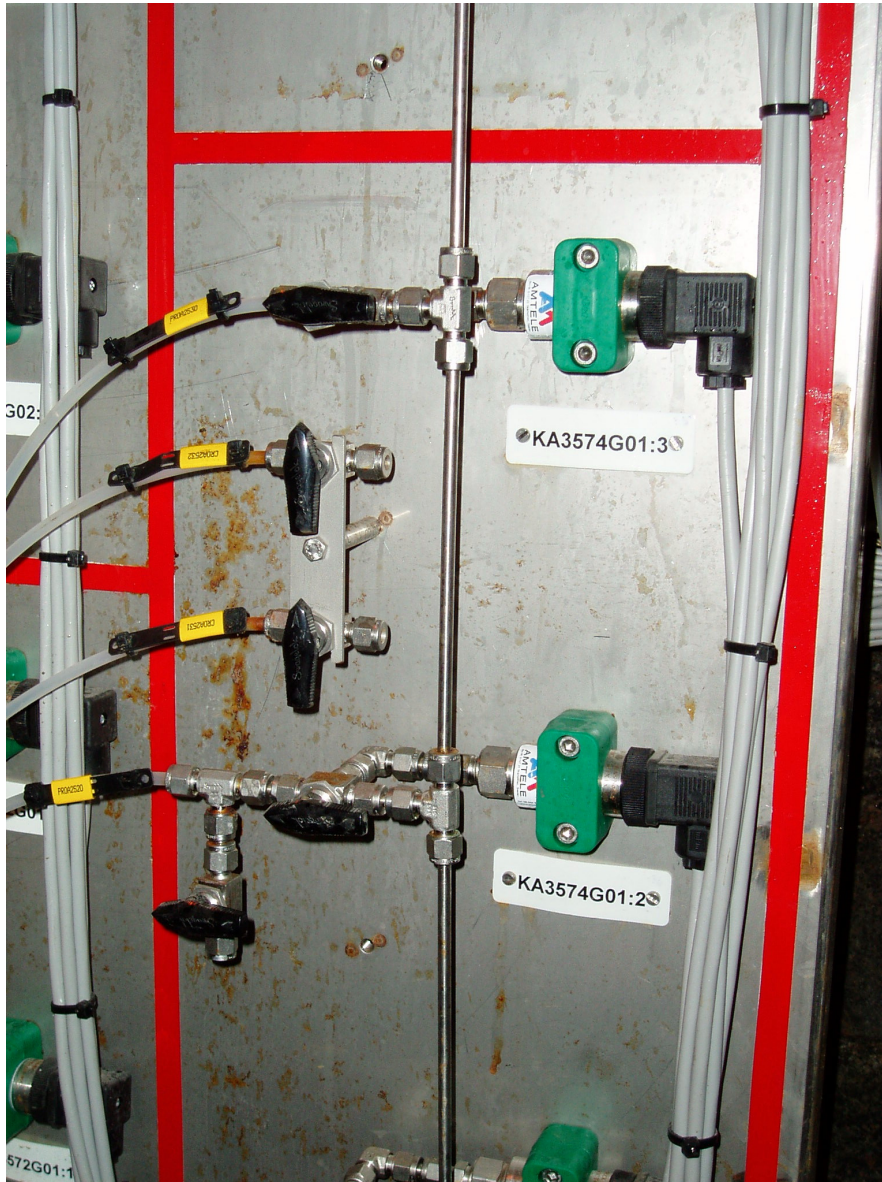
Figure 4-2. Pressure transducers connections
