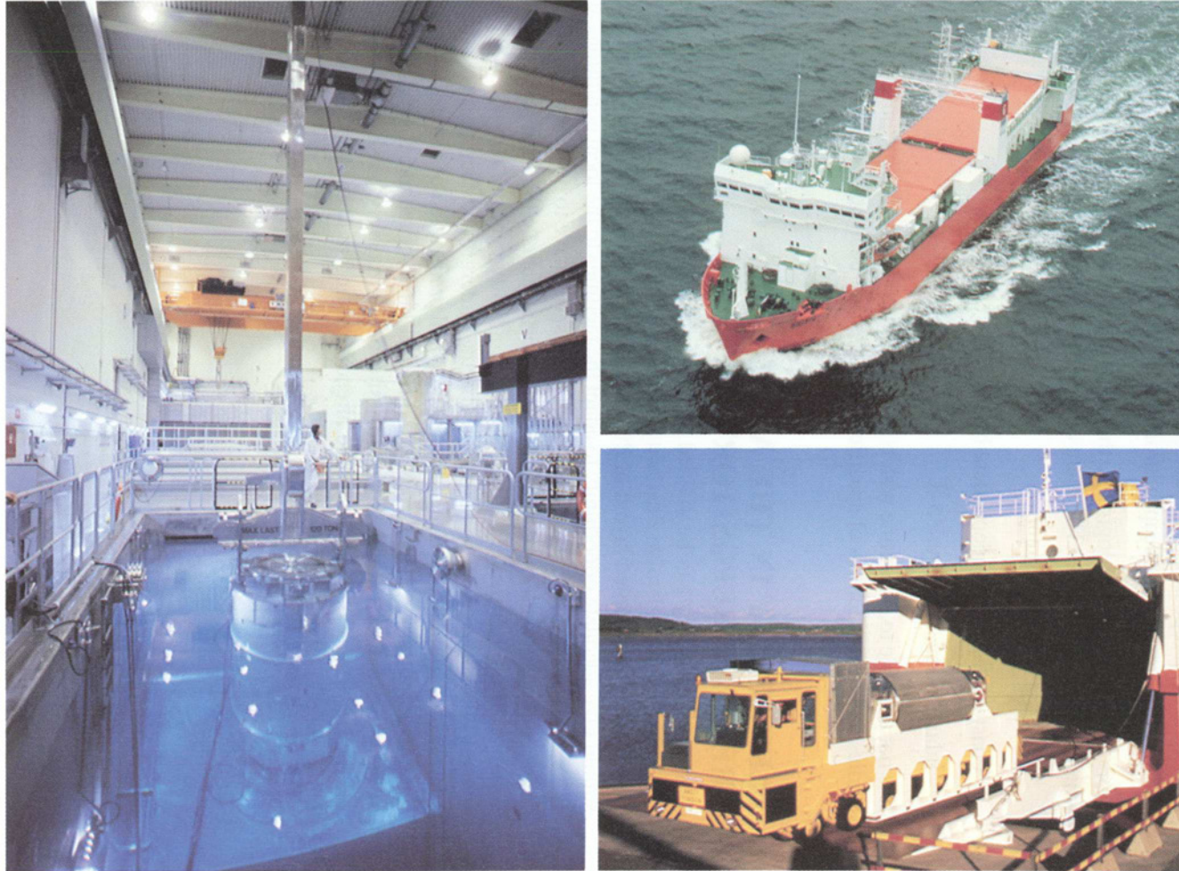
Figure 5-2 Spent nuclear fuel is stored for about 40 years in water-filled pools in the central interim storage facility for spent nuclear fuel (CLAB) at Oskarshamn. During this time, the radioactivity decays and the heat generated by the fuel is reduced by 90%, which allows for simpler handling of the fuel during encapsulation and transportation to the deep repository. However, since the level of radioactivity will still be high, the spent fuel will be transported in special containers similar to those currently used for non-encapsulated spent nuclear fuel. If the repository is located inland, a harbour terminal will be constructed for receiving and loading the fuel onto trucks or trains.
