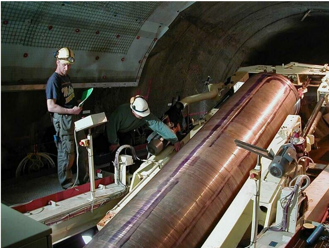
Figure 2-1 Deposition of a full scale canister in Äspö HRL.
