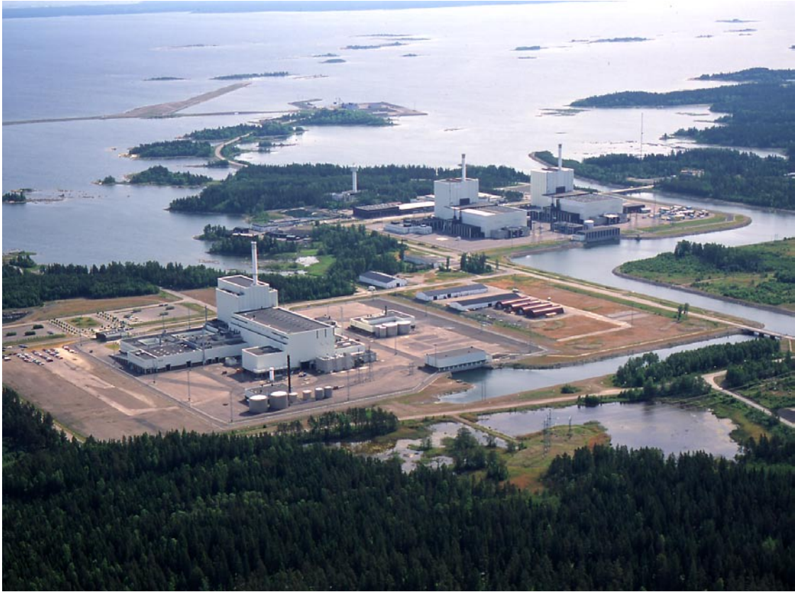
Figure 2-9. Industrial area in Forsmark, with the three reactor buildings, and in the background the SFR facility.
