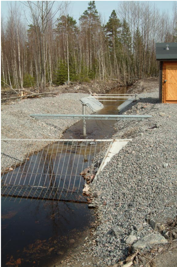
Figure A-8. Flow monitoring station upstream of Bolundsfjärden.
