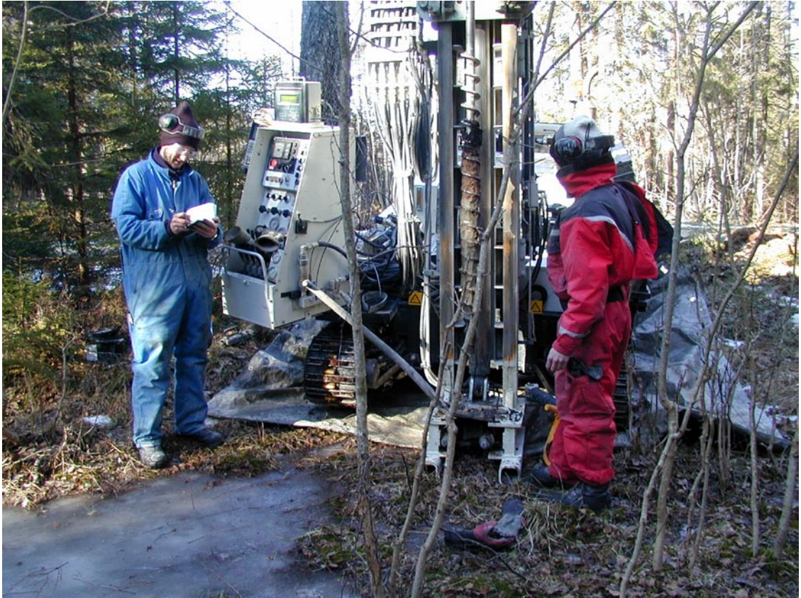
Figure A-6. Auger drilling machine.
