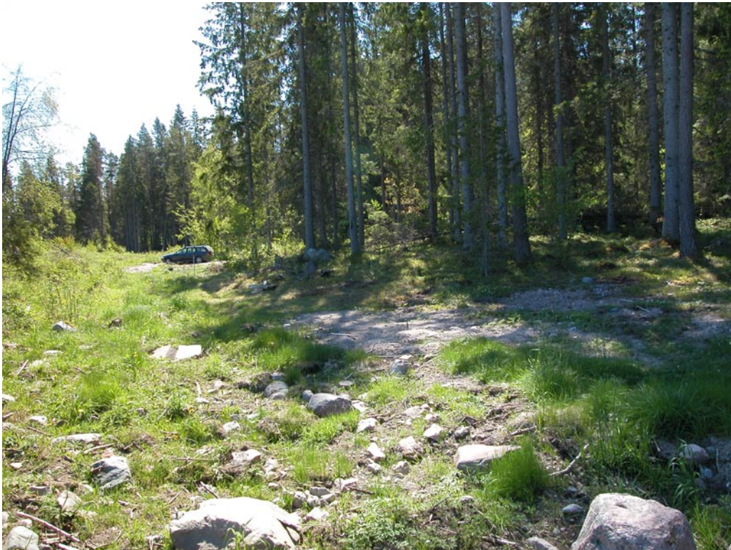
Figure A-3. Trench for Quaternary deposit mapping during and after excavation.
