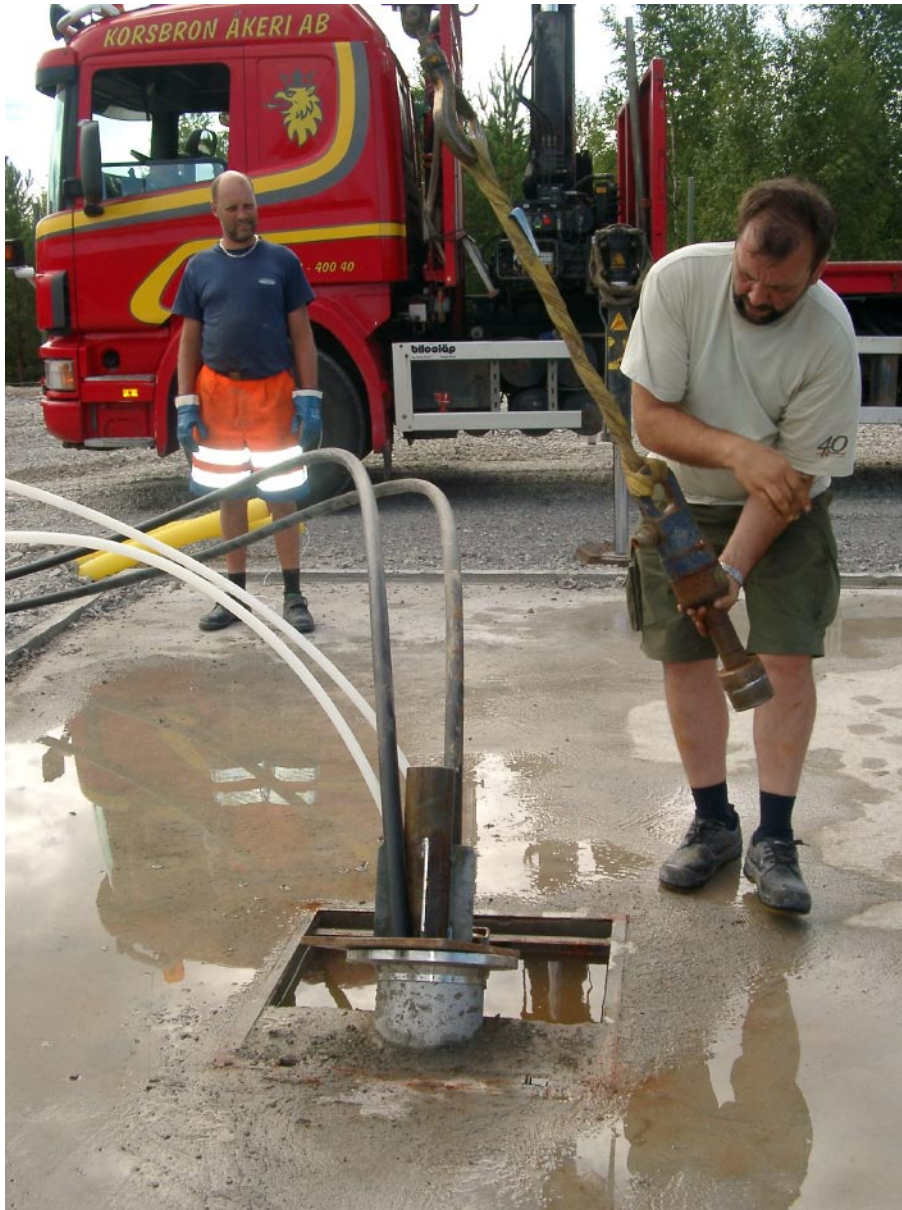
Figure 3-7. Installation of airlift pumping equipment in borehole KFM04A.
