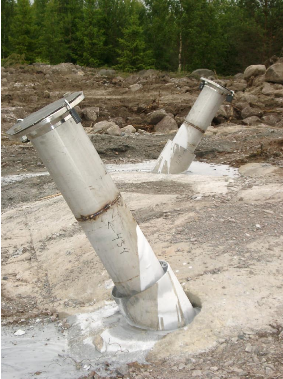
Figure 4-1. Boreholes KFM04A and KFM04B secured with lockable stainless steel flanges.
