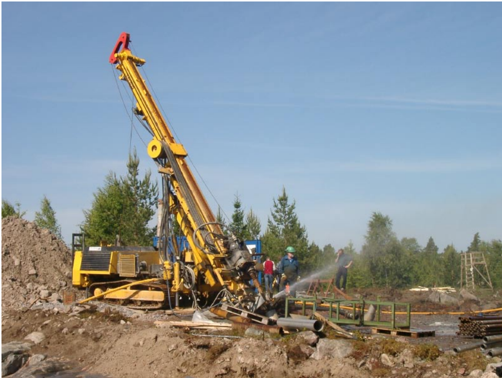
Figure 3-1. The Puntel drilling machine during drilling of KFM04A and KFM04B at drilling site DS4.
