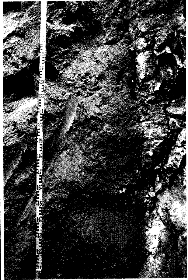
Fig. 11. The sharp, vertical contact between bedrock and till in the fault-zone at Molberget. Photo: R. Lagerbäck 1987.
