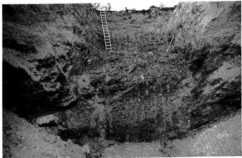
Fig. 15. The fractured and chemically weathered bedrock in the hanging wall at Stupforsen. The bedrock was easily cut through by the excavator. Photo: R. Lagerbäck 1987.
