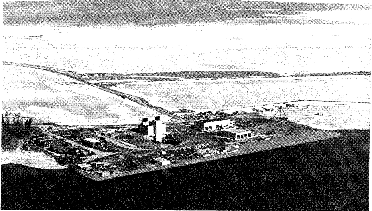
Figure 5-2. SFR – Overview of buildings on ground level.
