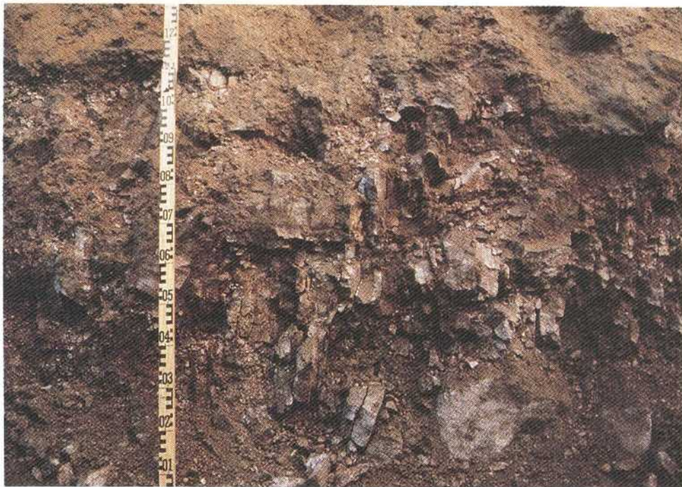
Figure 3-10. The fractured and chemically weathered bedrock in the hanging wall at Stupforsen. The bedrock was easily cut through by the excavator.
