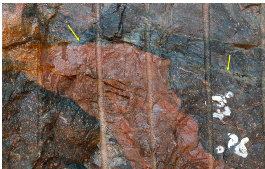
Figure 6-1. Localization of Structure #20 (yellow arrows) in relation to a dike of fine-grained granite exposed at chainage 76+00 in the TASS tunnel.
