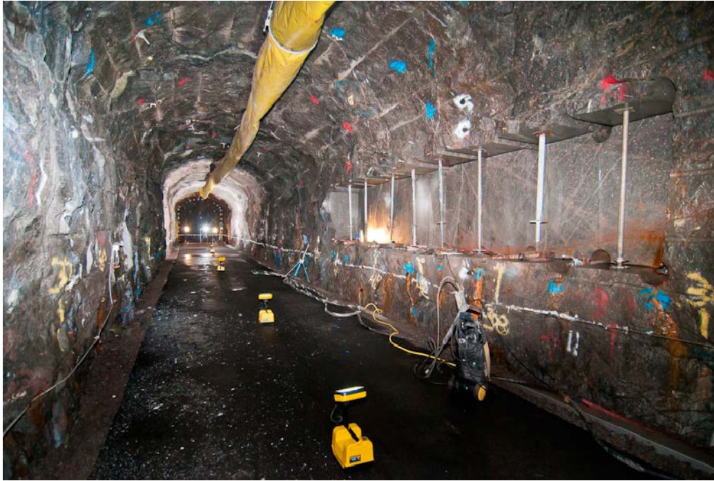
Figure 5-1. Wide-angle photograph of the TASS tunnel, illustrating portable construction lights used for site illumination. Note the lighted section near the end of the tunnel; this is the location of the Structure #20 intersection with the TASS tunnel. The elongated rectangular slot along right side of the tunnel wall is the excavation from the Excavation Damage Zone project (Olsson et al. 2009).
