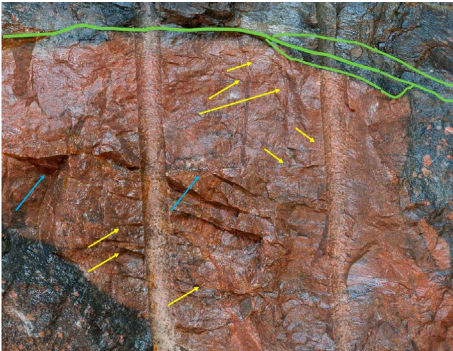
Figure 6-3. Close up of contact between fine-grained granite and Structure #20. Note the abundance of sealed fractures (yellow arrows) and partially open fractures (blue arrows) inside the fine grained granite. These fractures all have similar orientations to Structure #20, and are likely related to at least one phase of brittle deformation along the deformation zone. The green lines represent the open fractures inside the brittle core of Structure #20.
