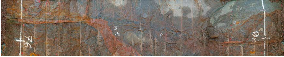
Figure 5-4. HDR image, after of a portion of the Structure #20 intercept within the TASS tunnel. This image has been extensively re-sized using Photoshop so as to fit into the report.
