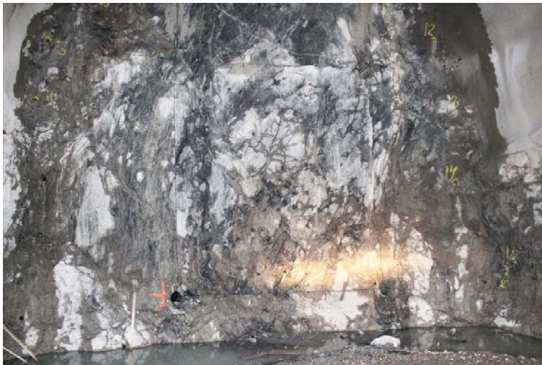
Figure A1-3. Photo of front pre-drilled before charging the round No 1.
