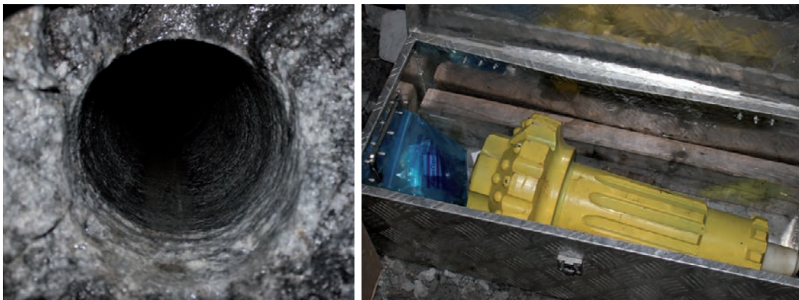
Figure 3-3. Photo of the reamed hole and drill bit used.
