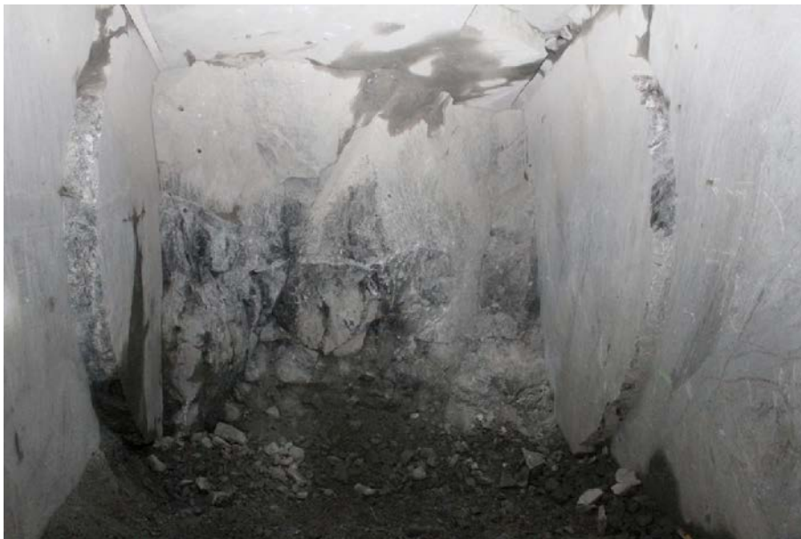
Figure 4-7. Photo of the face after blasting and loading of round No 4.
