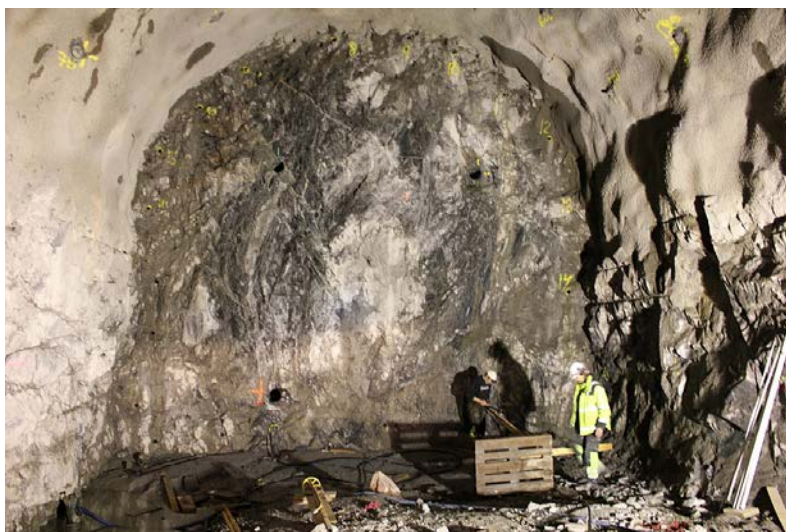
Figure 3-1. Photo of the front of the track tunnel with the four holes in the corners of the rectangular deposition tunnel drilled.
