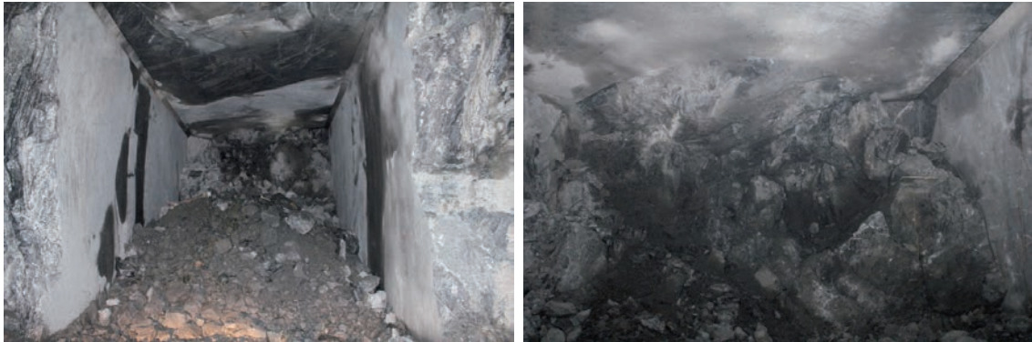
Figure 4-6. Photo of the face after the blasting of round No 3. The right figure shows also the residual crescent-shaped rock knob in the roof.
