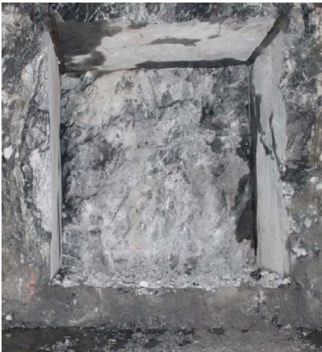
Figure 4-4. Photo of the face after blasting and loading of round No 1.
