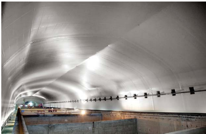
Figure 1-1. Rock vault for intermediate-level waste, 1BMA, in SFR.
