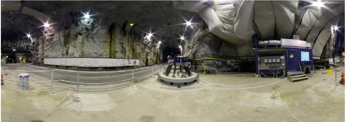
Figure 4-26. The Large scale gas injection test at the –420 m level in Äspö HRL.
