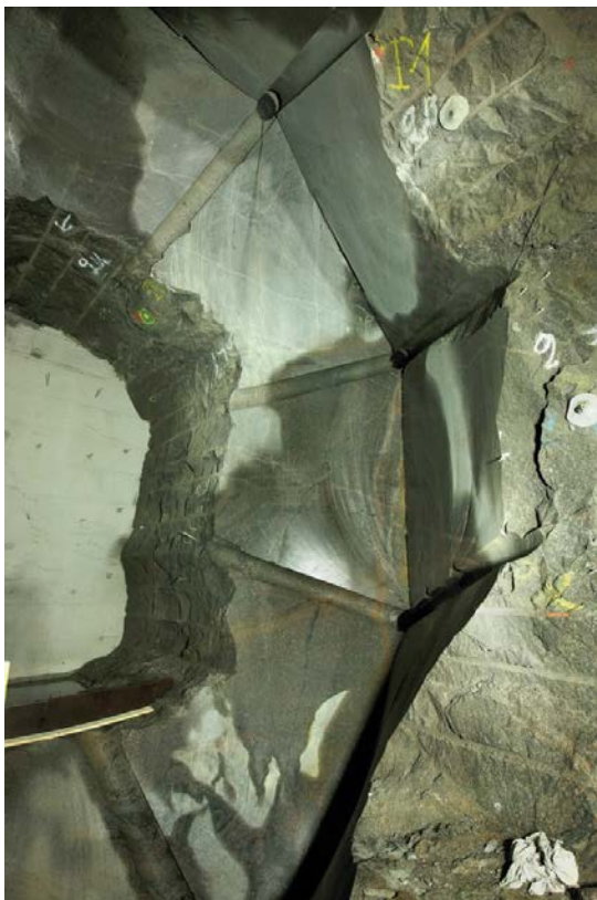
Figure 4-43. Part of the concrete dome abutment, excavated by wire-sawing.
