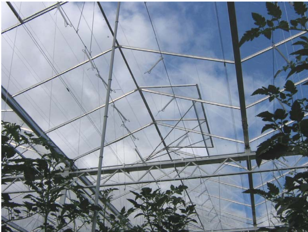
Figure 7-21. Interior view in a Venlo greenhouse with single glass as covering material. Photo: Sven Nimmermark.
