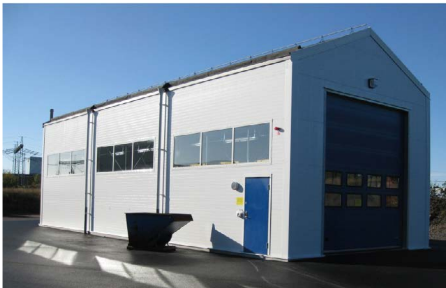
Figure 6-7. The new washing hall.
