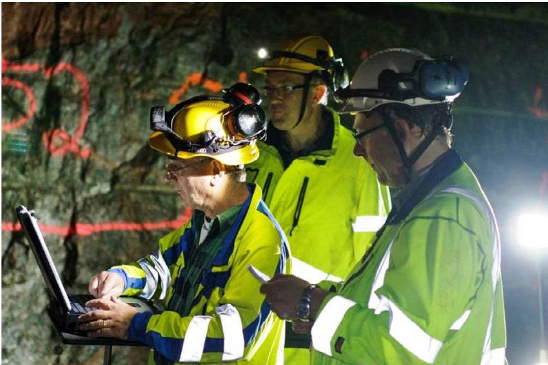
Figure 2-4. TASP-tunnel. Geological mapping with the RoCS system in tunnel environment.
