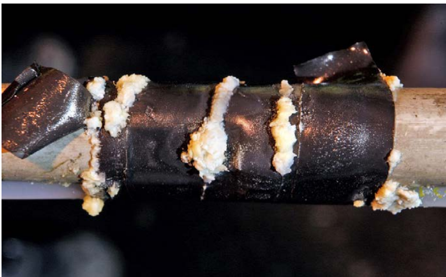
Figure 3-2. Pipe string of aluminium, plastic tubing and black tape. Precipitates of Al-oxyhydroxides and Si-rich precipitates. Corrosion of aluminium beneath tape.
