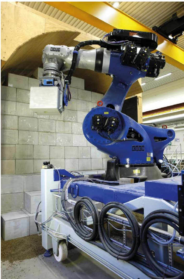
Figure 4-41. Industrial robot for backfill block installation.
