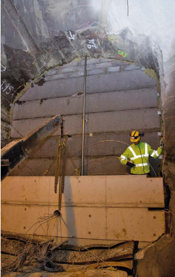
Figure 4-45. Installation of concrete delimiters, bentonite seal, macadam filter and sensors.
