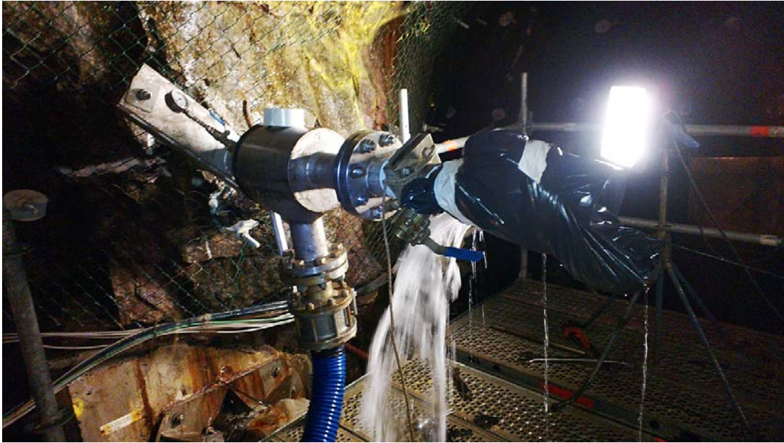
Figure 5-3. Outflow from the borehole at KA3065A01.
