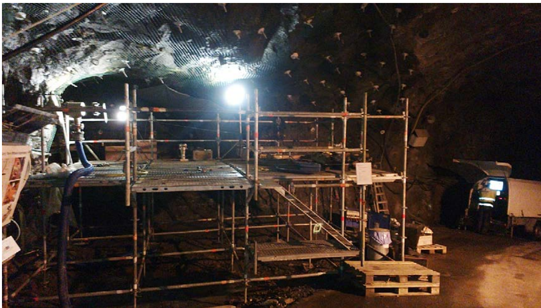
Figure 5-2. Measurement trailer mobilised at KA3065A01.
