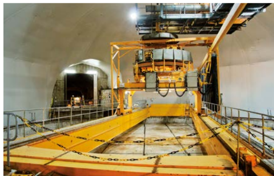
View over top of silo
