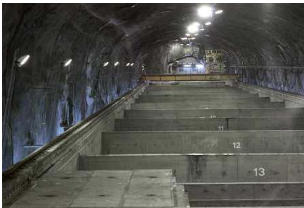
Figure 7-3. The rock cavern for short-lived intermediate level waste, 1BMA in SFR.
