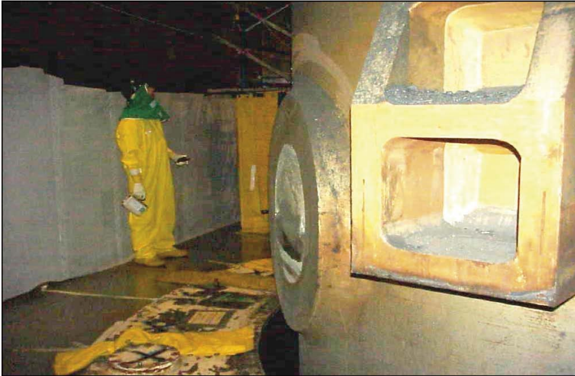
Figure A1-10. San Onofre Unit 1 Reactor Vessel Nozzles after cutting with a diamond wire saw.
