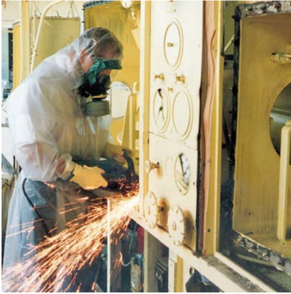
Figure 3-11. Typical manual plant dismantling operations.
