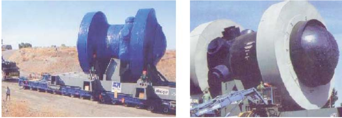
Figure 3-6. Views of Trojan Reactor Vessel with the radiation shield and impact reducers during transport.
