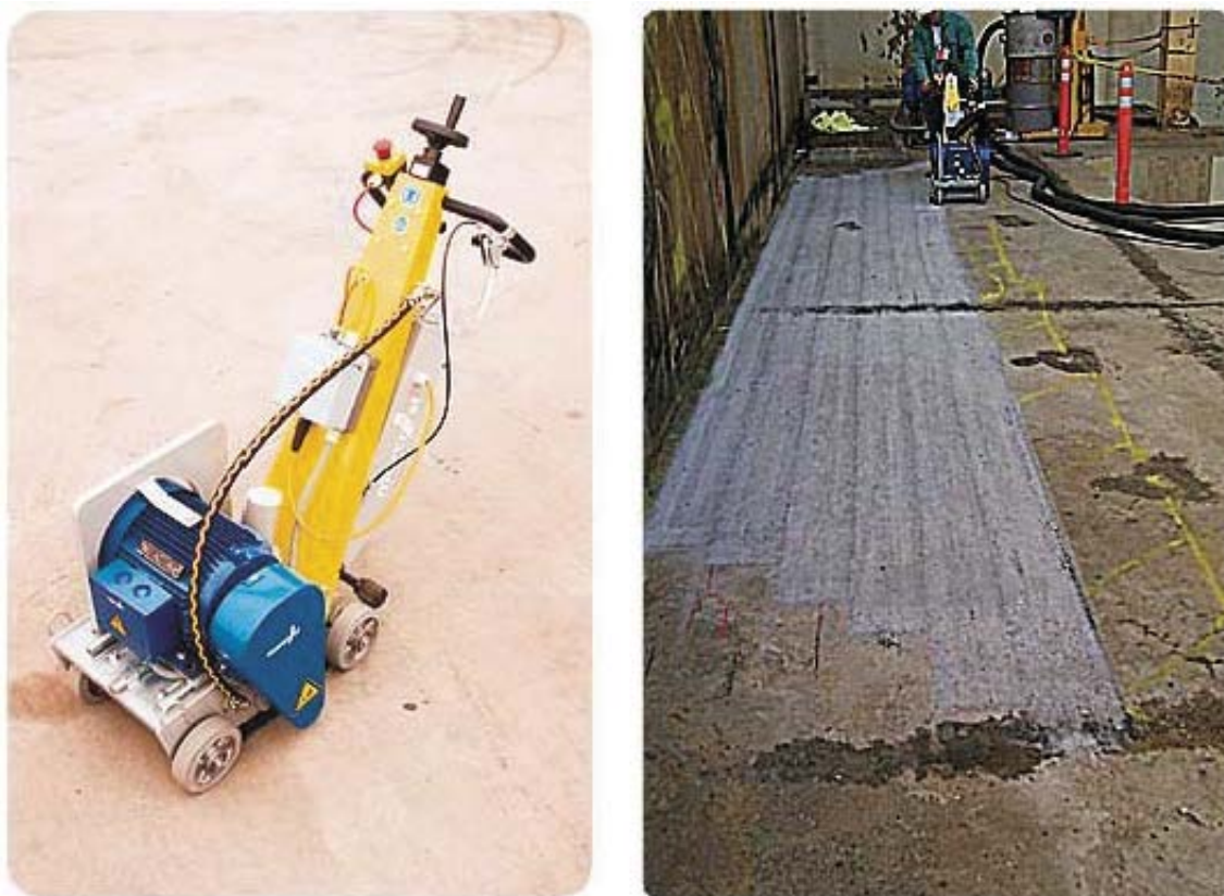
Figure A1-16. Marcris Floor Shaver and the resulting floor surface.
