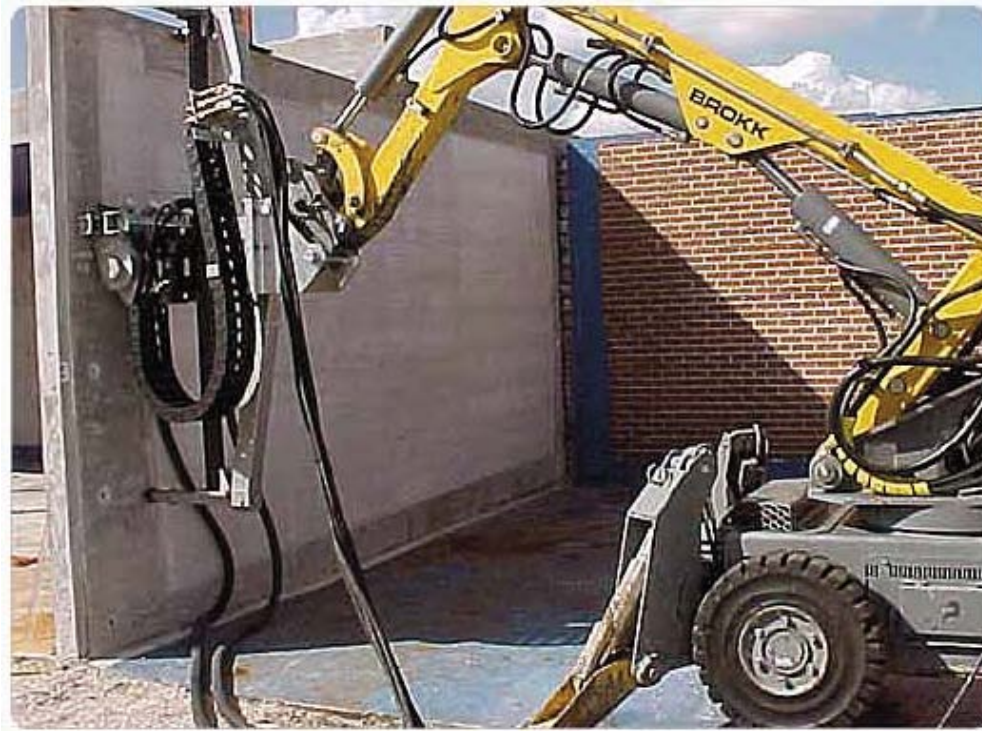
Figure A1-17. Floor Shaver mounted on Brokk 250 for wall decontamination.
