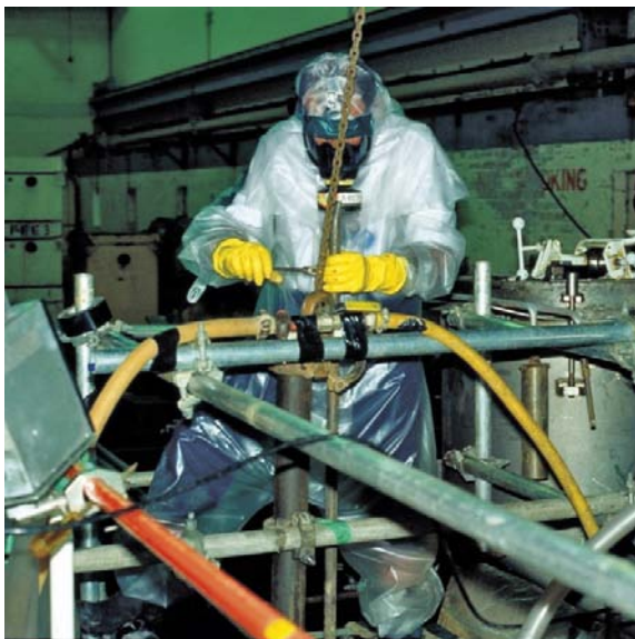
Figure 3-10. Preparation work prior to plant dismantling operations.
