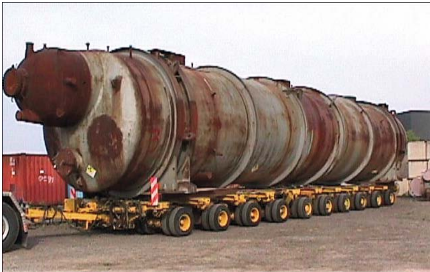
Figure A1-30. Re-heater transported from Oskarshamn 2.
