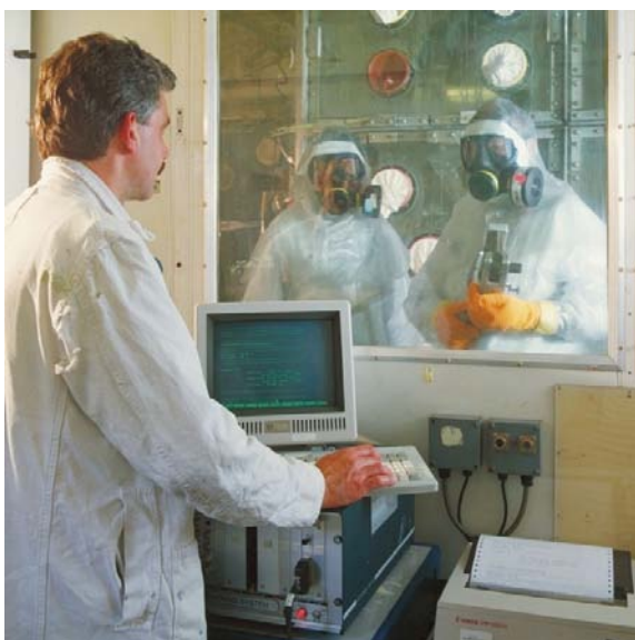
Figure 3-8. Manual dismantling operations utilizing Re-usable Modular Containment (RMC).
