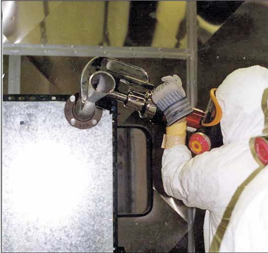
Figure A1-13. Mega Tech Blade Plunging Cutter being used to cut 2.5 inch OD pipe.
