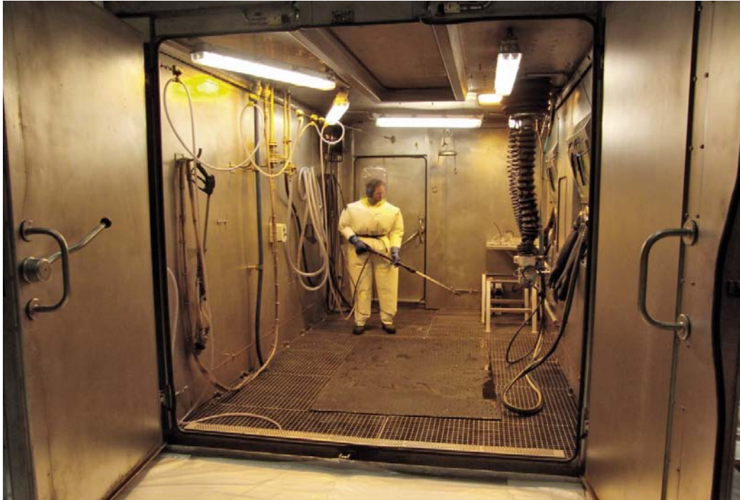
Figure 3-9. High pressure water decontamination facility at Forsmark.
