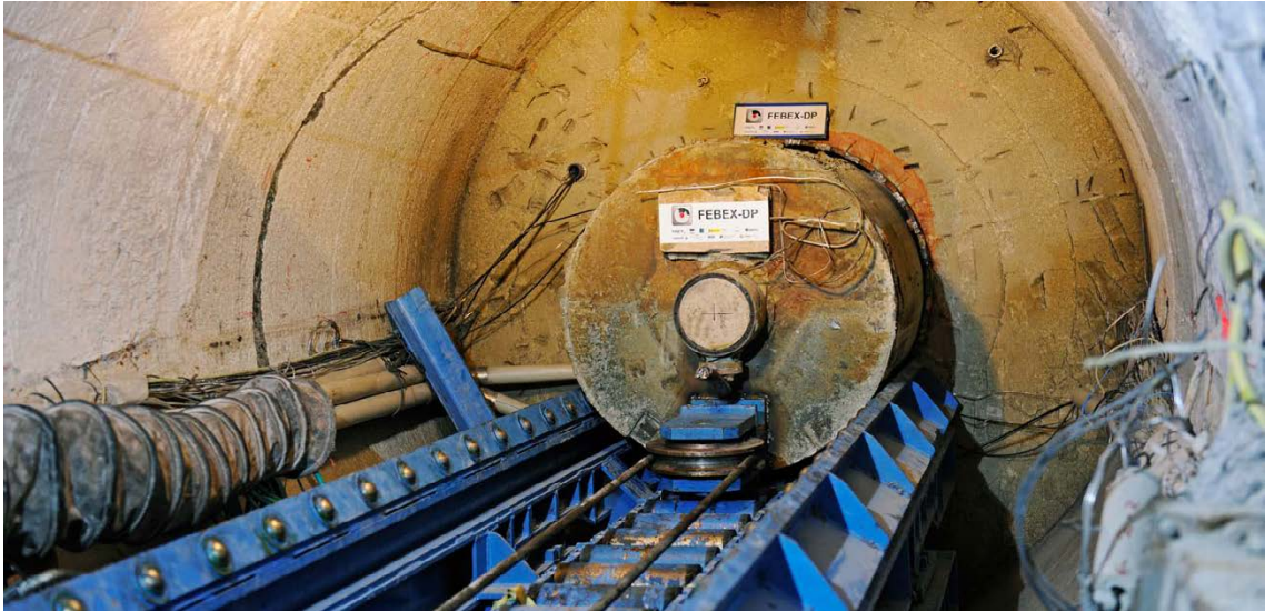
Figure 2-15. Extraction of Heater 2 during final dismantling (García-Siñeriz et al. 2016).
