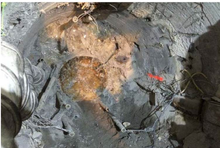
Figure B-5. View of the gallery after the dismantling of the shotcrete plug. The front of the 1 m long dummy steel cylinder that was placed during the first dismantling to fill the void left by heater #1 is visible. (García-Siñeriz et al. 2016).
