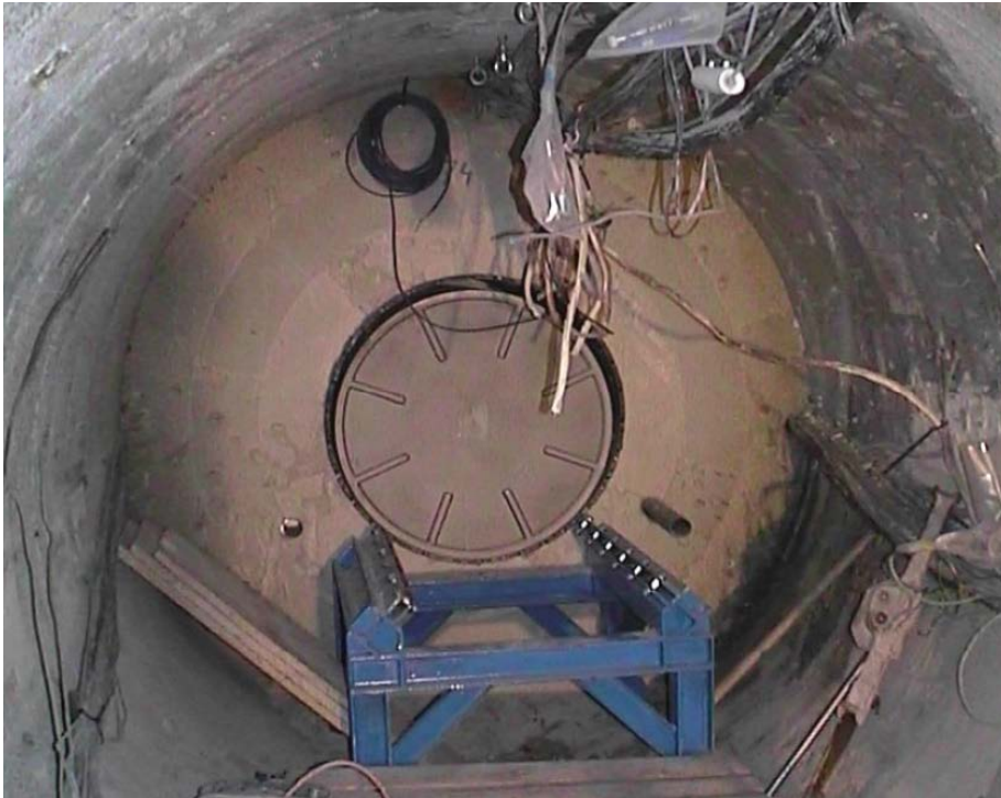
Figure A-42. Insertion of the dummy steel cylinder (Bárcena et al. 2003).
