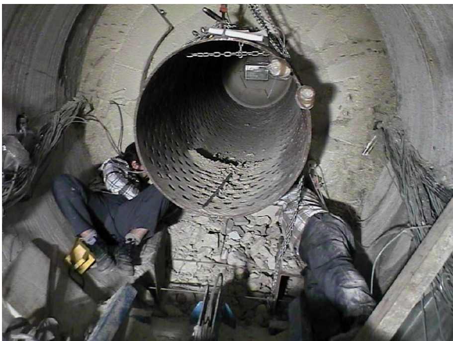
Figure A-41. Dismantling works in the heater section (Bárcena et al. 2003).
