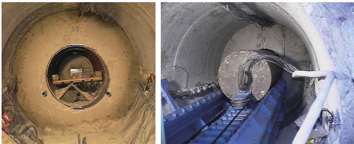
Figure 2-12. Left: State of the barrier after 5 years of heating. Right: Extraction of heater #1 during the first dismantling (Barcena et al. 2003).
