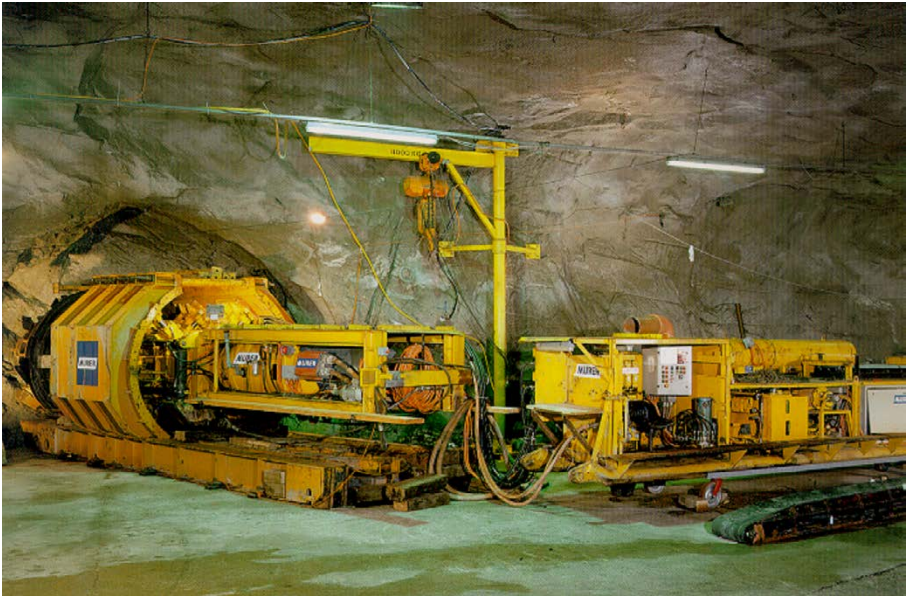
Figure 2-4. Excavation of the FEBEX experiment tunnel.
