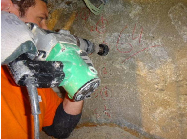
Figure B-8. Samples extraction with core drill (García-Siñeriz et al. 2016).
