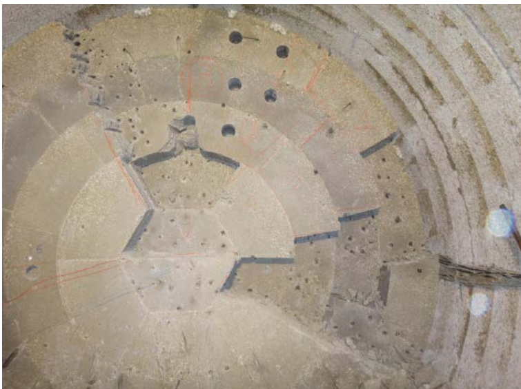
Figure B-9. Partial dismantling of a section (García-Siñeriz et al. 2016).
