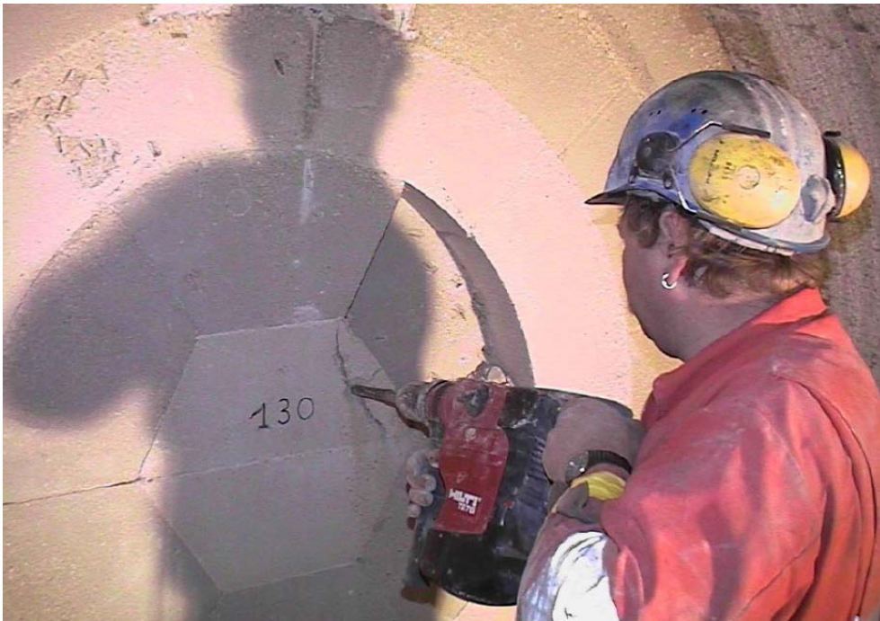
Figure A-39. Dismantling of bentonite layers (Bárcena et al. 2003).
