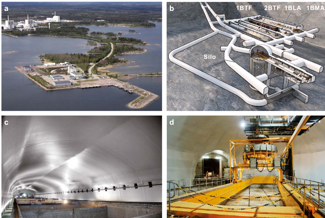
Figure 2-2. The final repository for short-lived radioactive waste (SFR) consists of two waste vaults for concrete tanks (1–2BTF), a waste vault for low-level waste (1BLA), a waste vault for intermediate-level waste (1BMA) and a silo for intermediate-level waste. a) View of the surface facility, b) SFR underground, c) waste vault, d) View of silo top.
