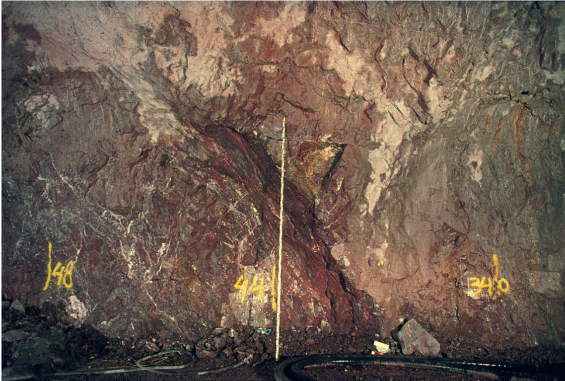
Figure 4-7. Clay-filled fracture in brecciated metagranite within the core of the Singö Deformation Zone in the Forsmark 1 and 2 tunnels as described in Carlsson and Olsson (1977). Photo G Hansson/N.
