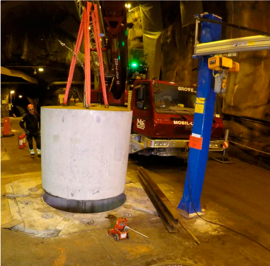
Figure 15-18. Lift of the concrete plug using a crane.
