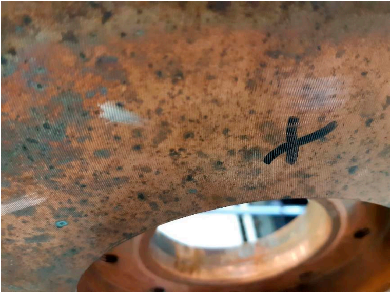
Figure 3-96. Close-up of area of the canister base, with dark patches near the position of PC901.
