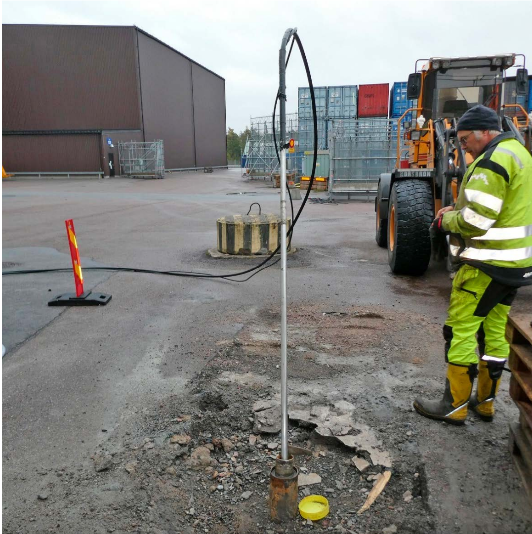
Figure 5-6. The mammoth pump with two hoses (one for the air supply and the second for return water) ready to be lowered into borehole KFM27.
