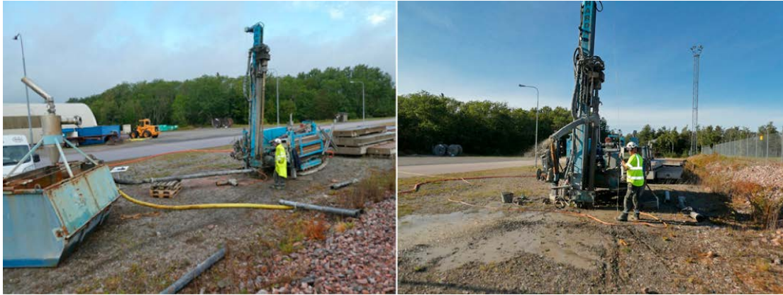
Figure 5-10. Right. The HARDAR 5000H drilling machine at drill site HFM47, close to the VEGA office. Left. With a total water-inflow of only c. 6 L/min it is difficult to clean the borehole from drilling debris after completed drilling. For effective flushing it was therefore necessary to add water in order to get the borehole cleaned.
