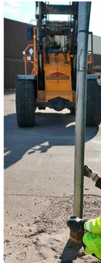
Figure 5-4. Left: As monitoring boreholes probably will be used for several decades, the inner casing is made of acid proof stainless steel. Right: The casing is lowered into the outer casing, and is centralized by three steerings for every three metres casing length.
