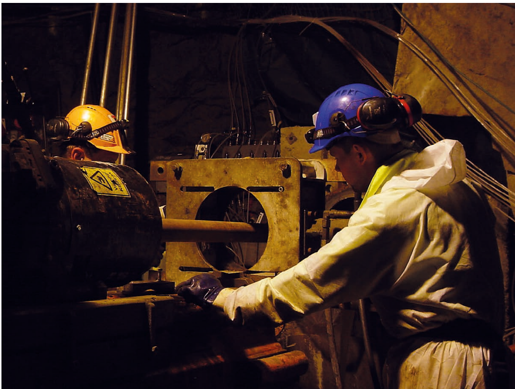
Figure A7-6. Supervising drilling.
