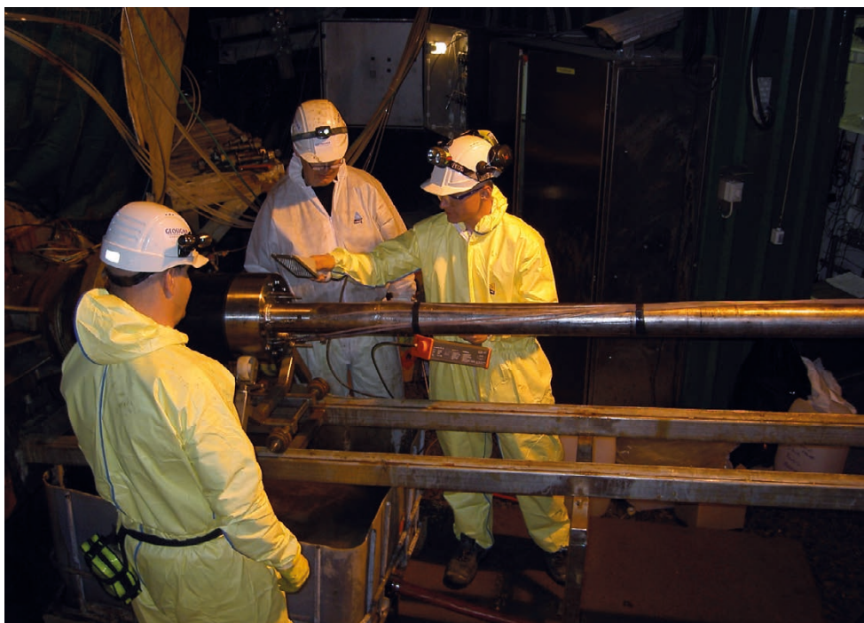
Figure 2-8. Measurement of radioactivity by scintillation detector during the procedure of removal and dismantling.
