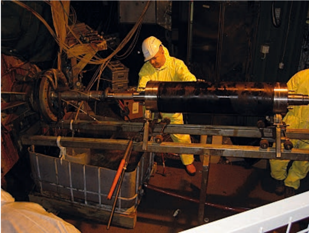
Figure A6-5. Hydraulic packer being disconnected from outer pipe.
