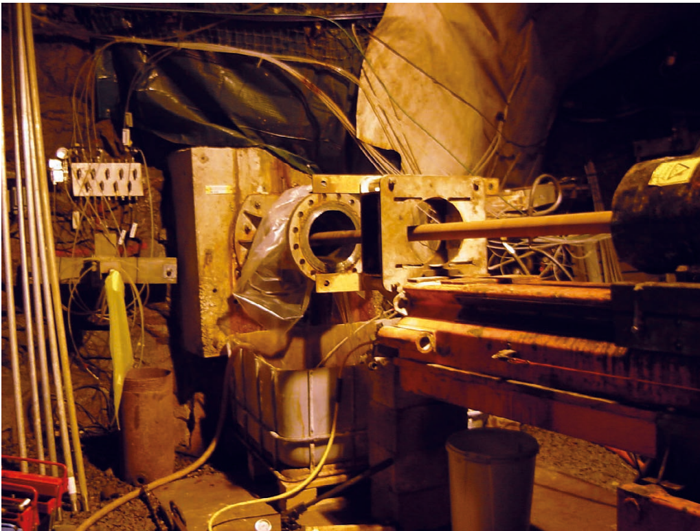
Figure A7-4. Ongoing over-core drilling. Drill pipe and drilling machine.
