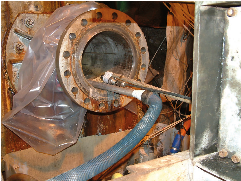
Figure A7-17. Borehole is drained by suction pump and inspected with borehole camera before start of drill phase 2.
