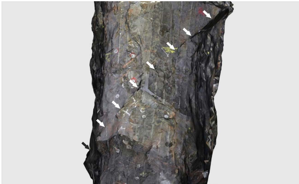
Figure 1-5. An example of a fracture with a full perimeter intersection, the TASS tunnel, Äspö HRL. View of the tunnel roof, based on a photogrammetric compilation.
