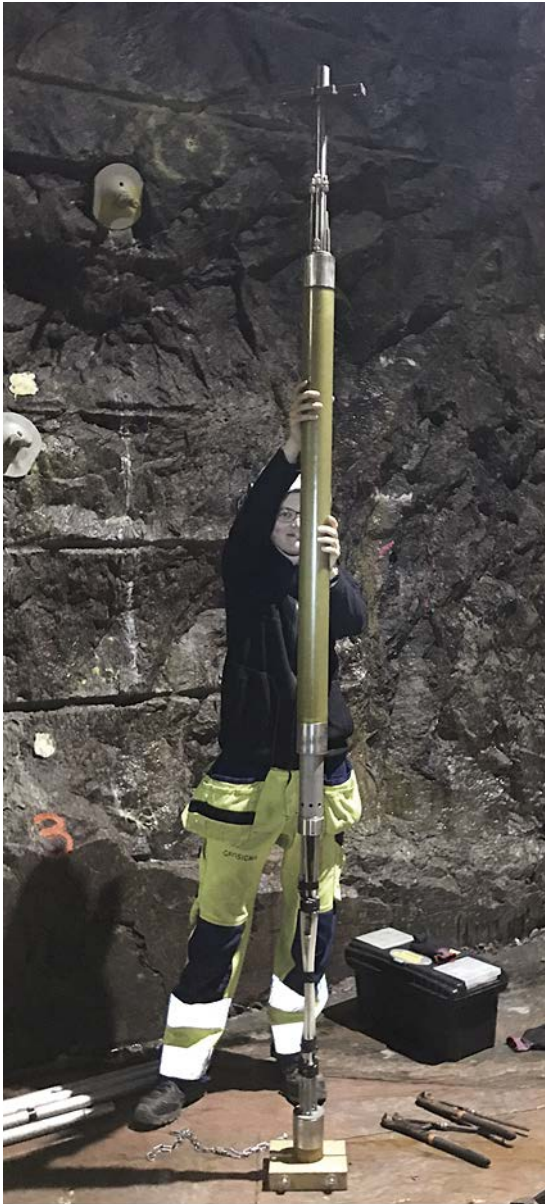
Figure 3-3. Installation of a double-packer for hydraulic tests.
