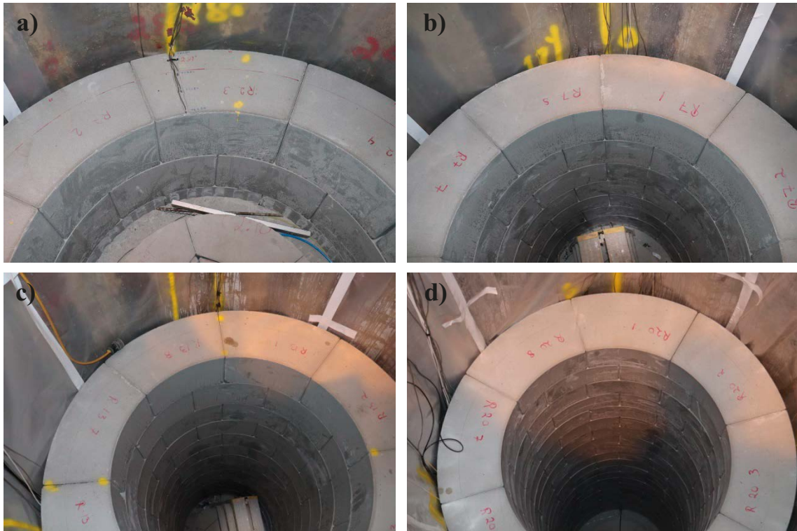
Figure 3-9. Installation of ring layers . a) R2, b) R7, c) R13, d) R20.
