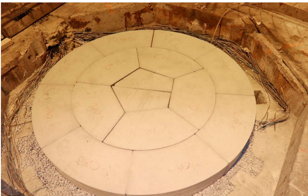
Figure 3-14. All blocks, pellets and instrumentation installed.
