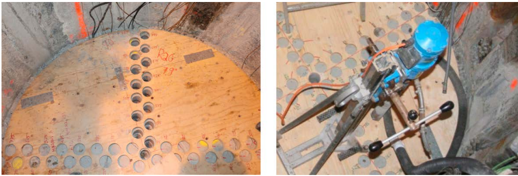
Figure 3-25. Left: Wood template used when core drilling. Right: Core drill.
