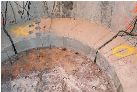
Figure 3-29. Layer R20 after the special centre blocks are removed.
