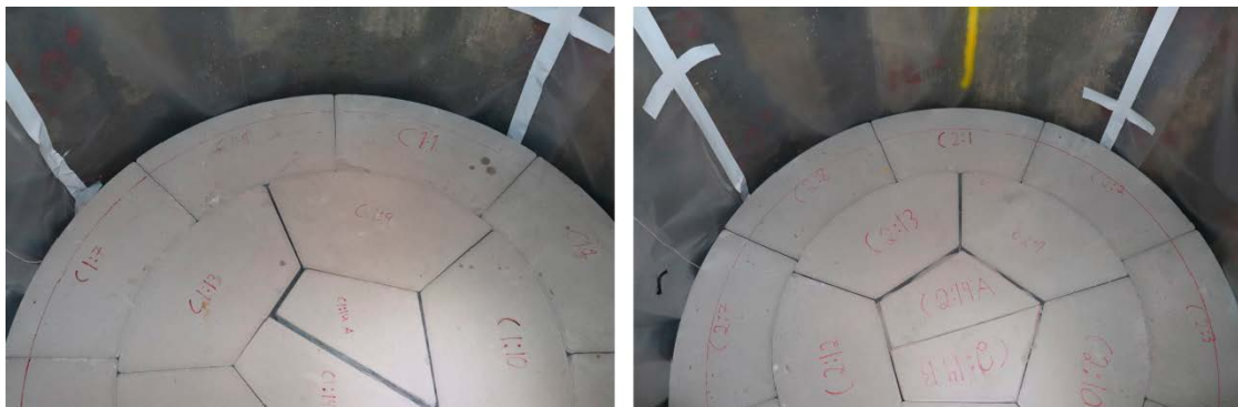
Figure 3-6. Installation of bottom layers. Left: layer C1, right: layer C2.
