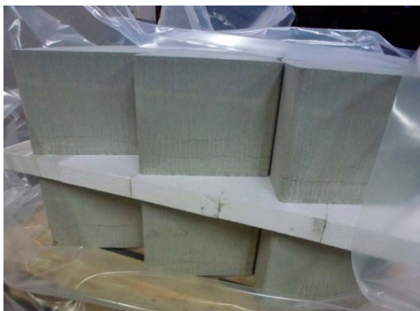
Figure 2-7. Euro-pallet with blocks. Small horizontal cracks can be seen on the lower half of the blocks.
