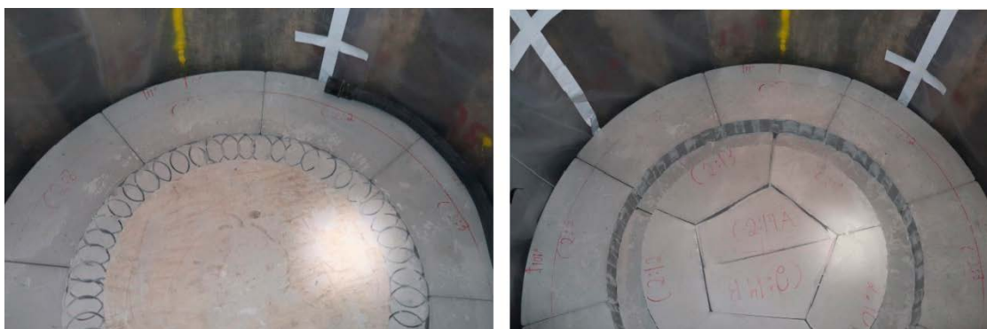
Figure 3-8. Left: Core drilling of slot in layer C2, right: Finished slot.
