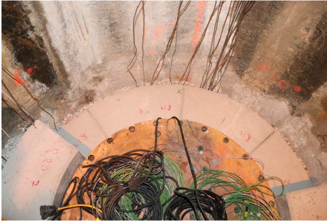
Figure 3-13. Removal of three damaged bentonite blocks.
