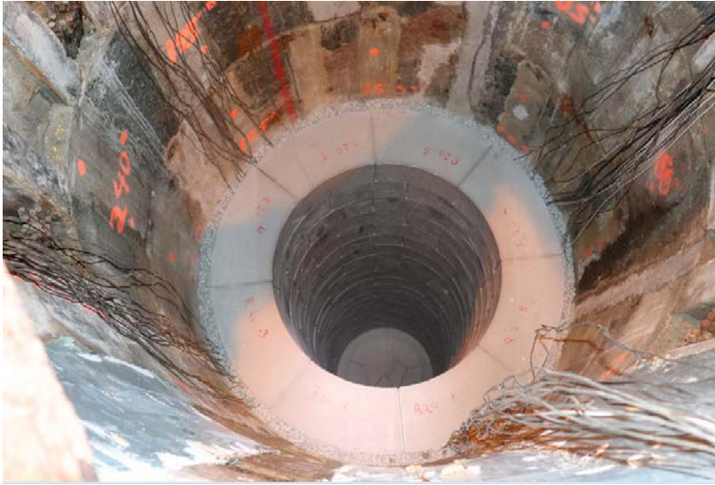
Figure 3-7. Buffer blocks and pellets installed to the canister's top level.
