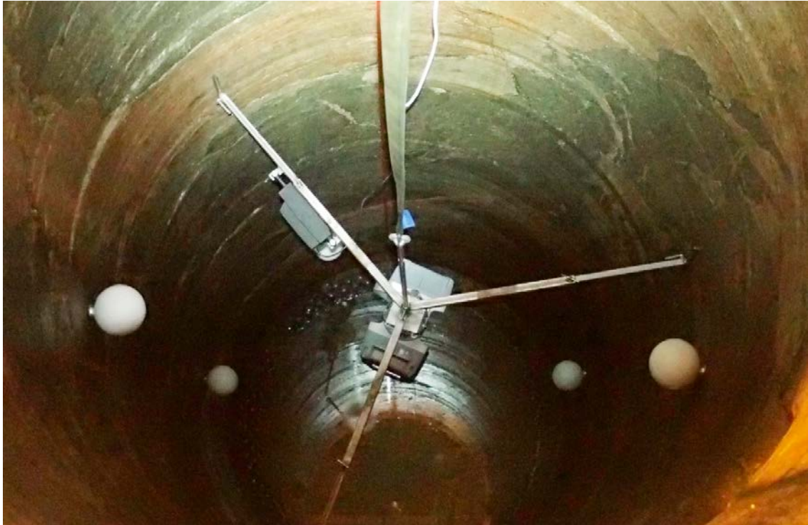
Figure 3-10. Scanning of deposition hole DO0010G01 with a Trimble TX8 Laser mounted on a fixable tripod rig to minimize instrumental vibrations.
