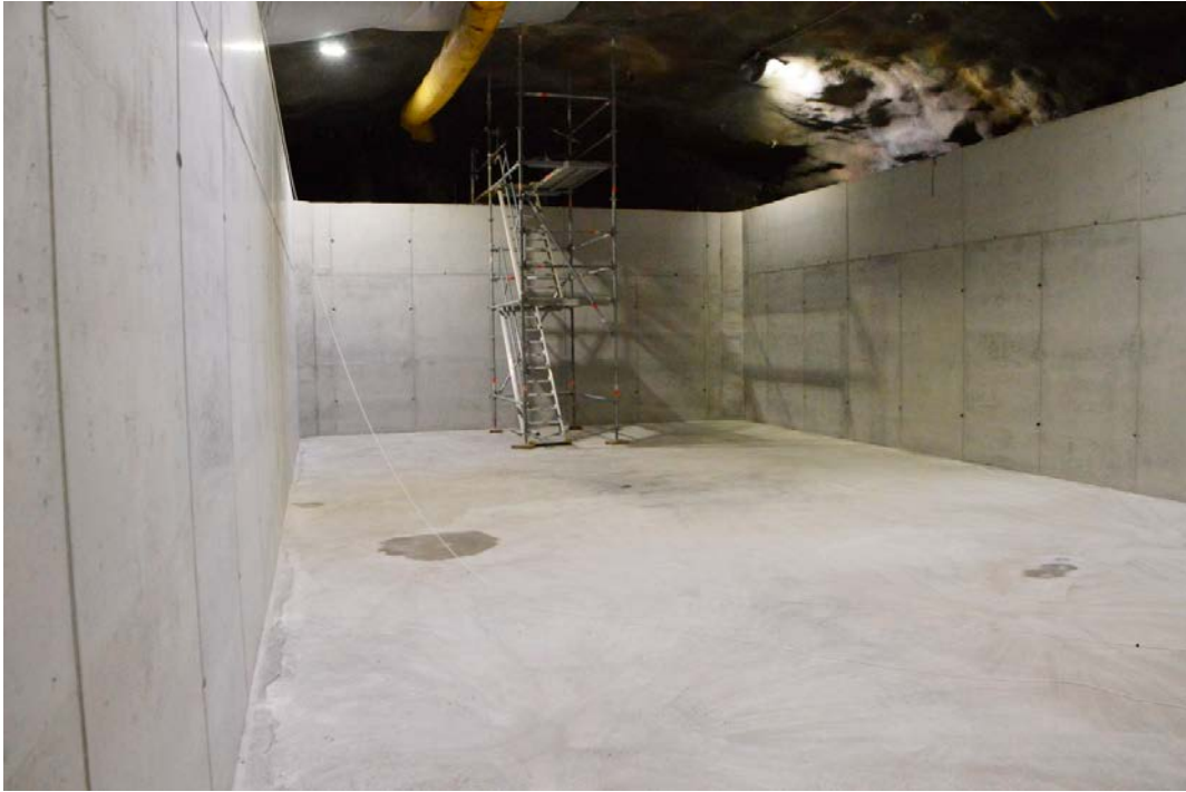
Figure 3-13. The interior of the concrete caisson after dismantling of the formwork.
