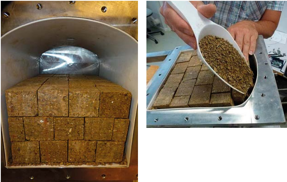
Figure 3-3. Photos taken during the installation of the backfill in the simulated deposition tunnel.
