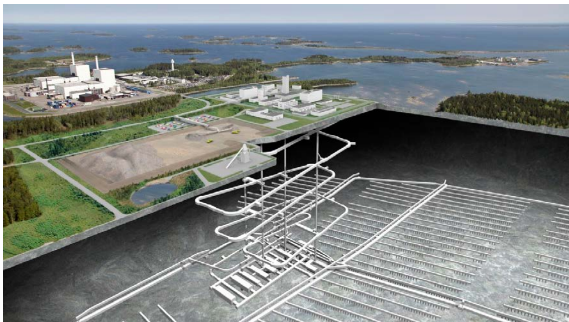
Figure 1-1. Planned deep repository for spent nuclear fuel, SFK, in the Forsmark area.
