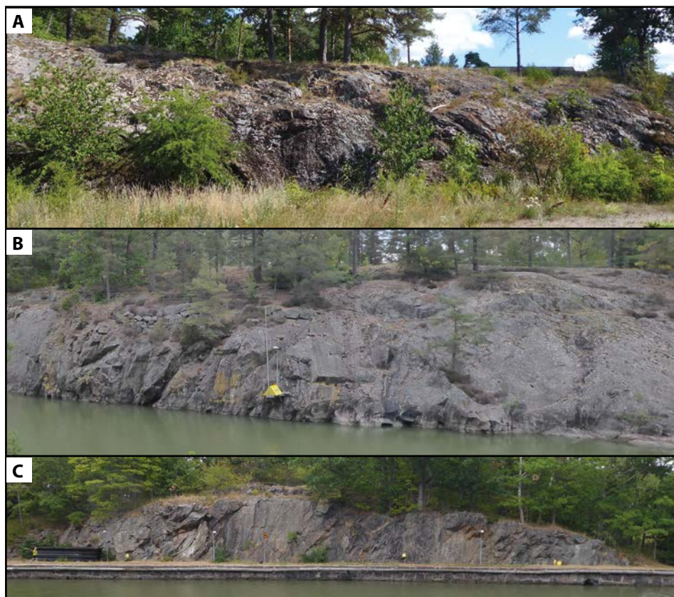
Figure 3-37. Sections aligned N-S along the Karls grav viewed from Rosenlund between Onsjö and Restad (Figure 3-14). A. Former quarry showing prominent fractures inclined to the NW and with NE-SW strike. B. Canal cut with curved sheet joints. C. Canal cut with fractures inclined to the NW. Planar flats occur on the highest ground on either side of the canal.
