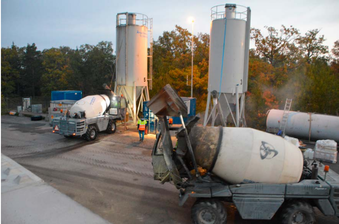
Figure 7-9. The concrete plant in full production.
