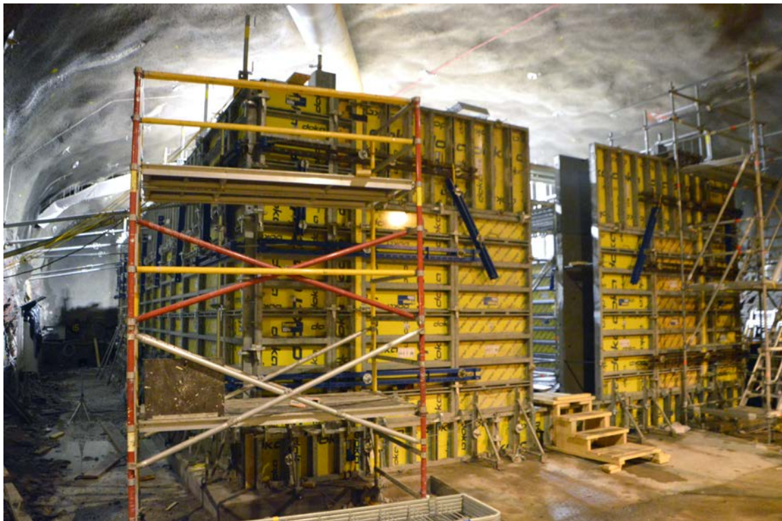
Figure 8-1. An overview image of the formwork just prior to completion.
