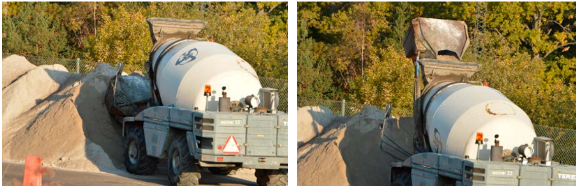
Figure 5-10. Feeding aggregates (0–4 mm) into the truck mixer.
