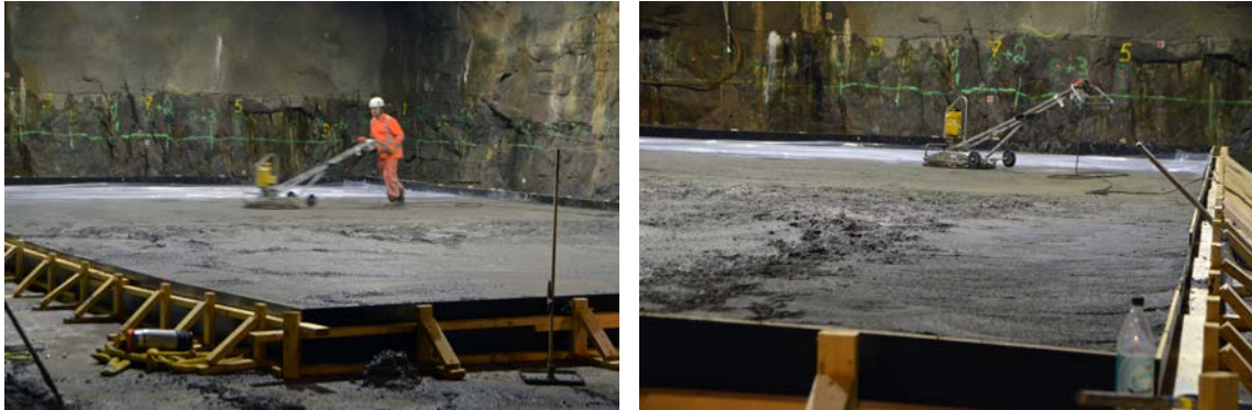
Figure 4-6. Trowelling of the concrete slab.
