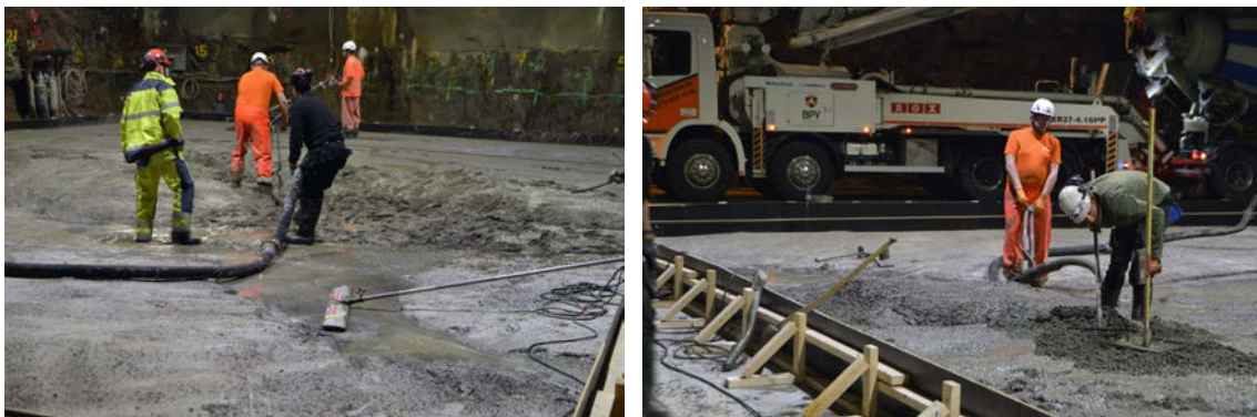
Figure 4-5. Casting of the top layer of the slab.
