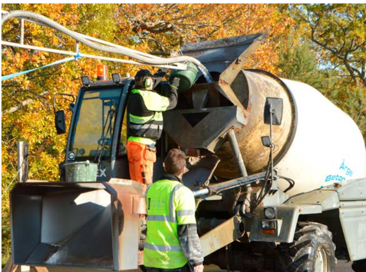
Figure 5-9. Feeding water and admixtures (in the bucket) into the truck mixer.
