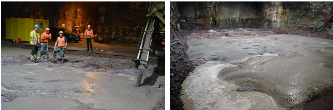
Figure 4-3. Filling of the largest pits in the outer part of TAS08.
