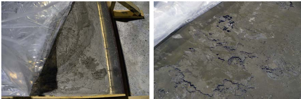
Figure 4-7. Surface finish of the trowelled concrete.
