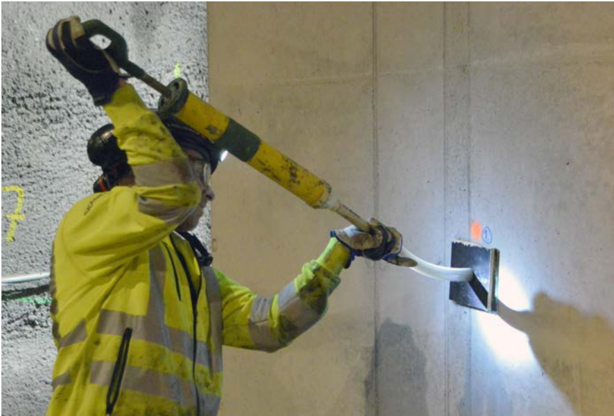
Figure 9-6. Grouting the hole with a hand-held injection pump.
