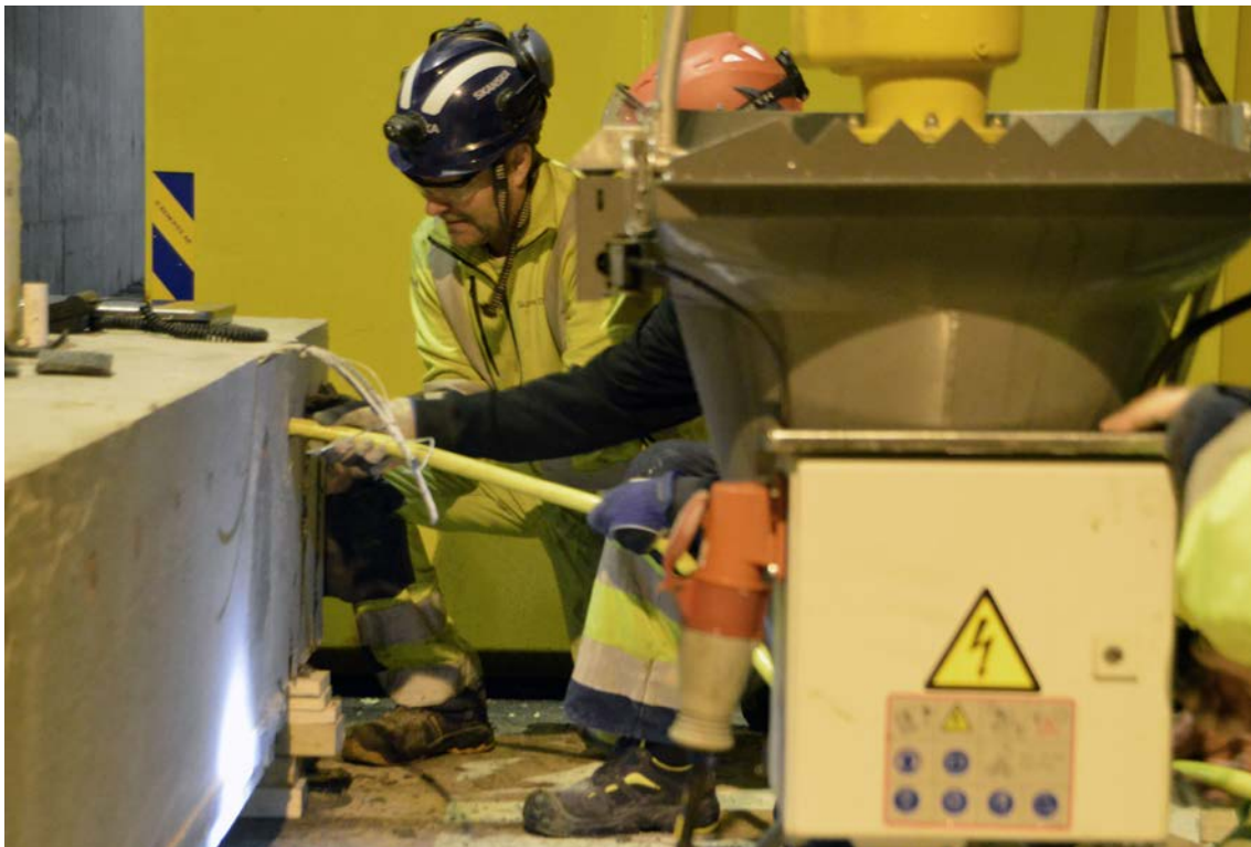
Figure 9-20. Grouting.
