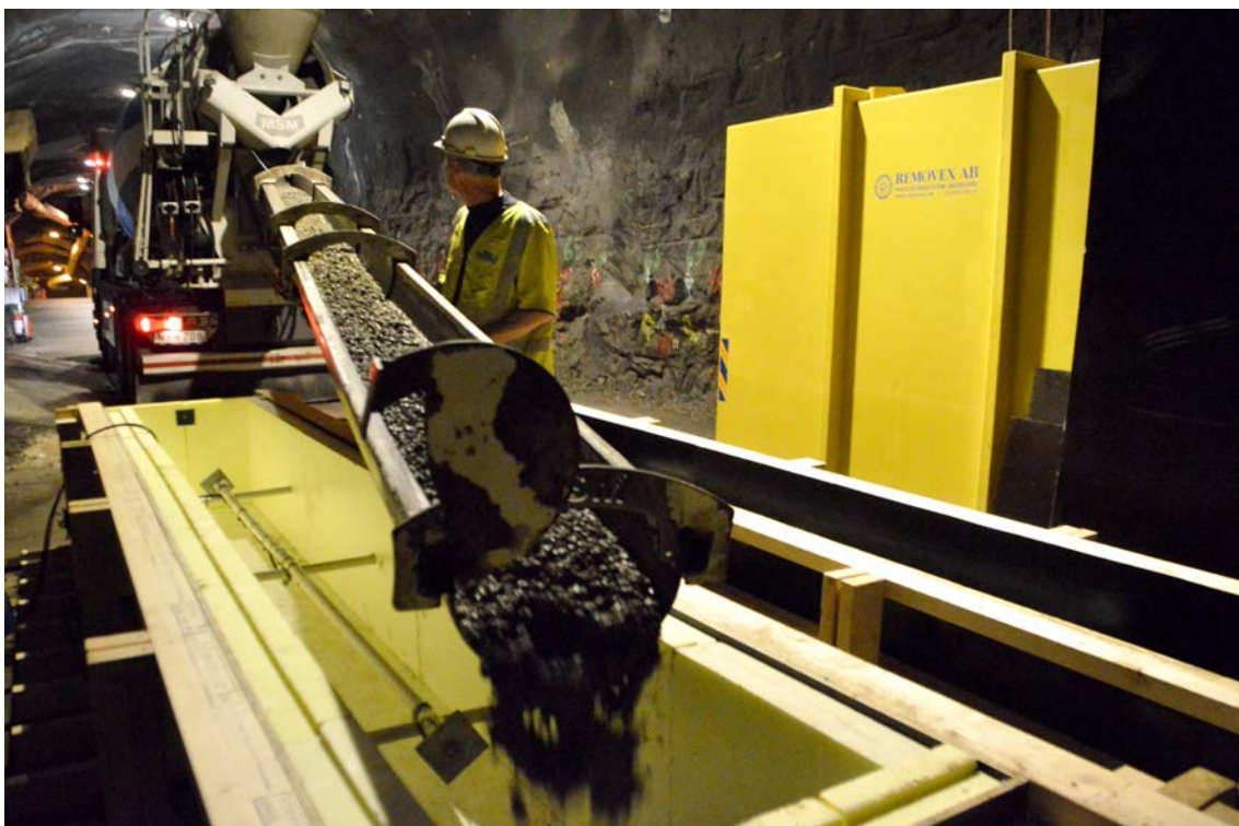
Figure 6-6. Casting of the beams using standard concrete.
