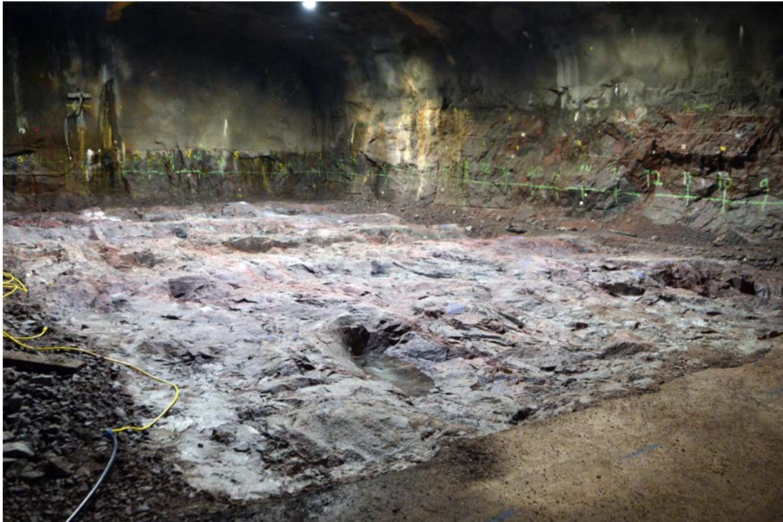
Figure 4-2. All rock debris in TAS08 has been removed and the bare rock exposed.
