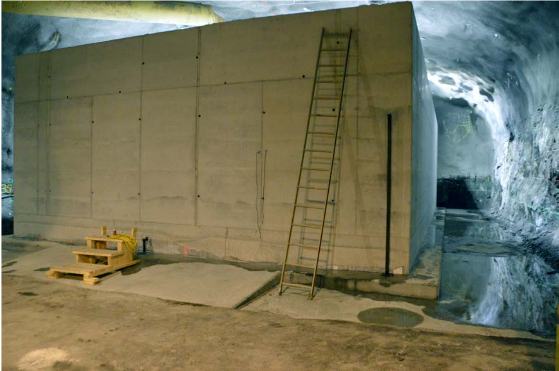
Figure 8-12. The caisson after dismantling of the formwork.
