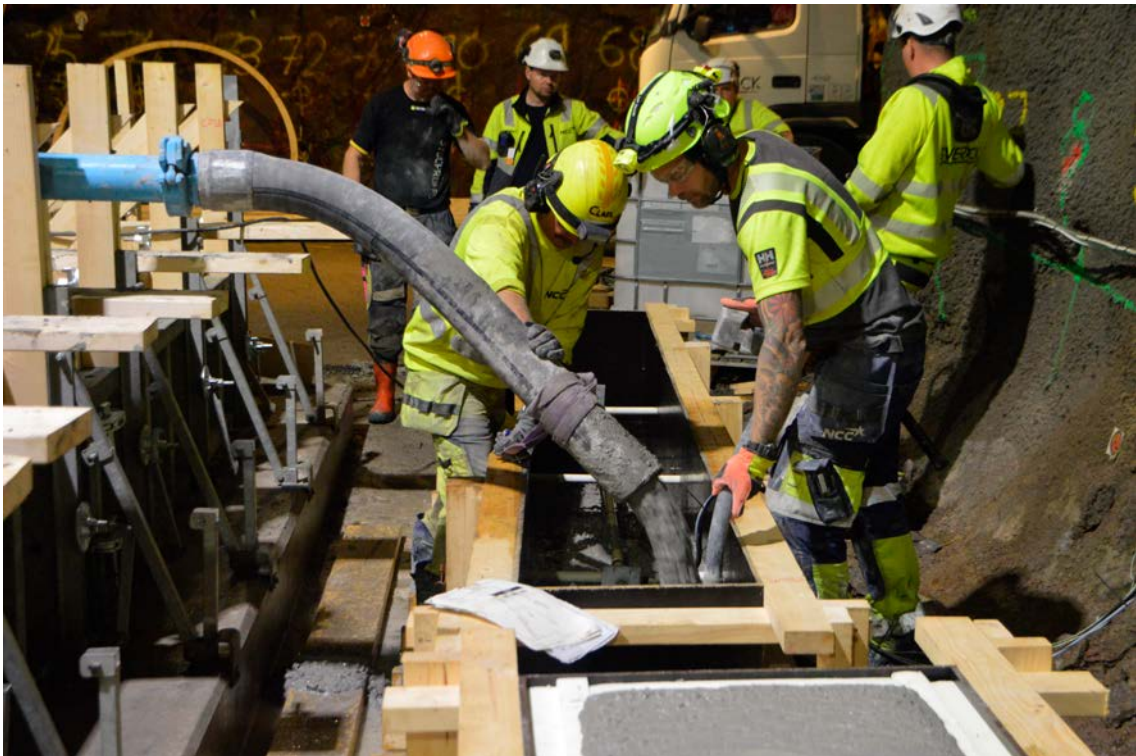
Figure 6-1. Casting of the beams using 2BMA concrete.
