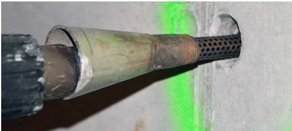
Figure 9-11. The hot air gun and perforated steel tube used to heat the plastic tube prior to extraction.
