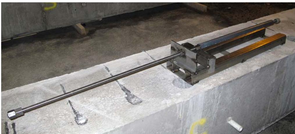
Figure 9-12. The extraction tool used to extract the plastic tubes from the concrete walls.
