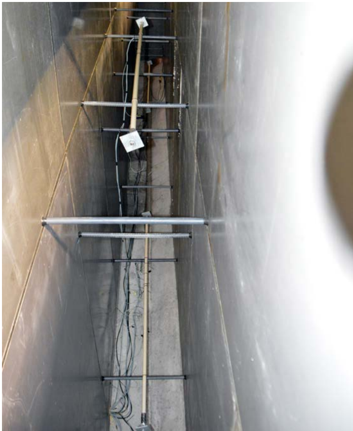
Figure 8-5. Strain transducers mounted in the form rods inside the formwork.
