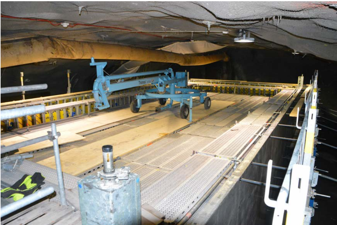
Figure 8-3. The concrete distributor has been lifted onto the platform.
