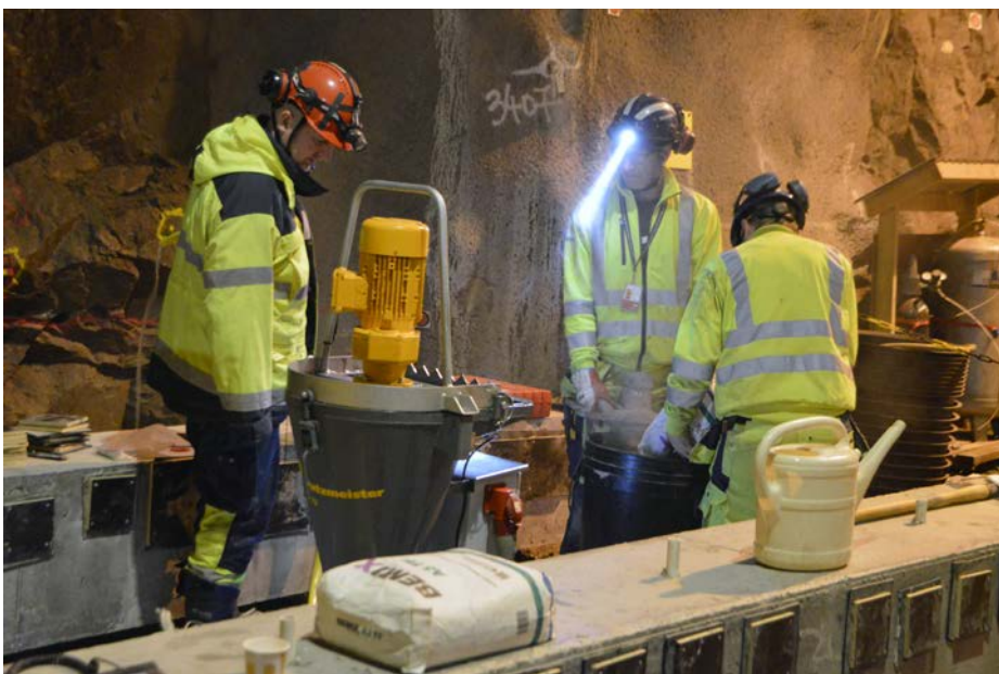
Figure 9-19. Mixing of grout.
