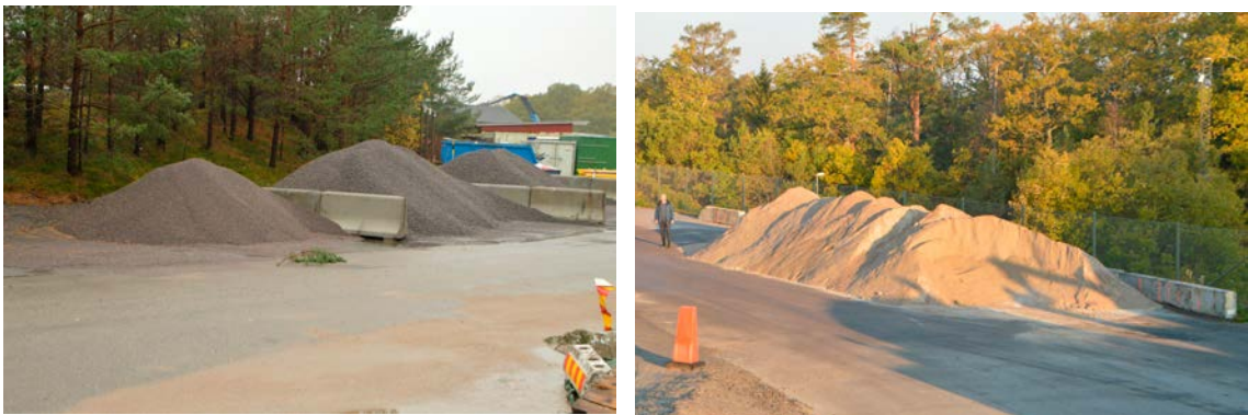
Figure 5-5. Storage areas for the 4 different aggregate fractions.
