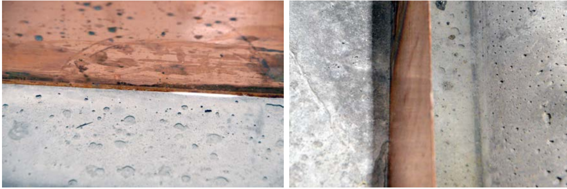
Figure 7-20. The joint seal cast into the base slab.
