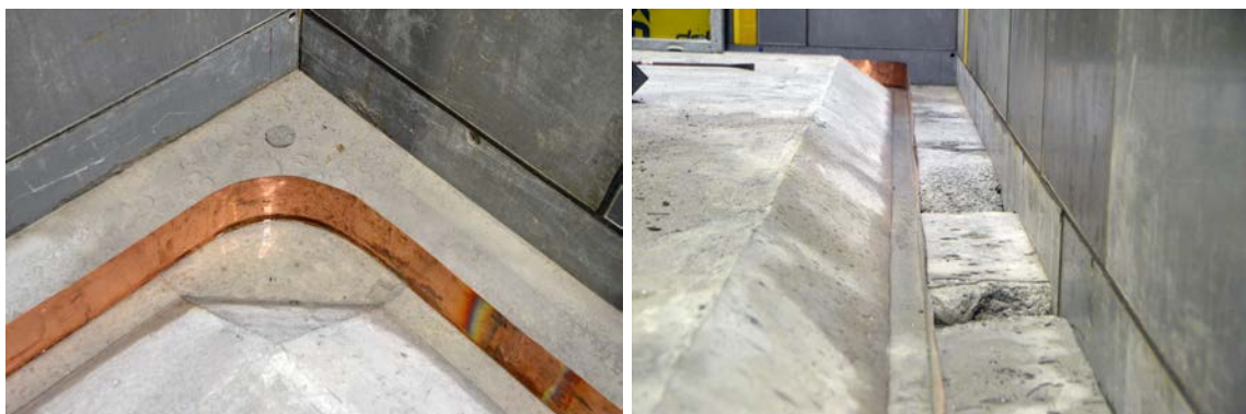
Figure 7-19. Images showing the joint against the walls in more detail. Note some positions with poor fill.
