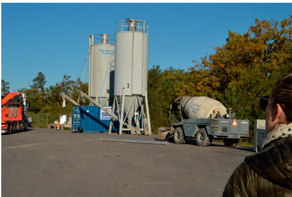
Figure 5-2. The two silos, each with a capacity of 50 tonnes.
