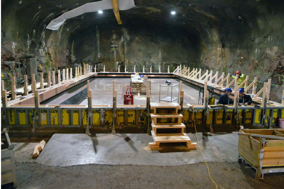
Figure 7-2. An overview picture of the formwork for the base slab.
