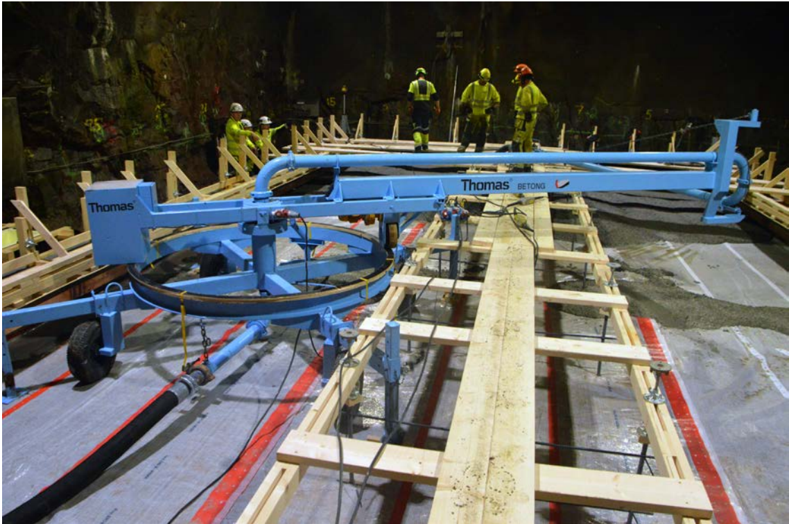
Figure 7-11. The concrete distributor.
