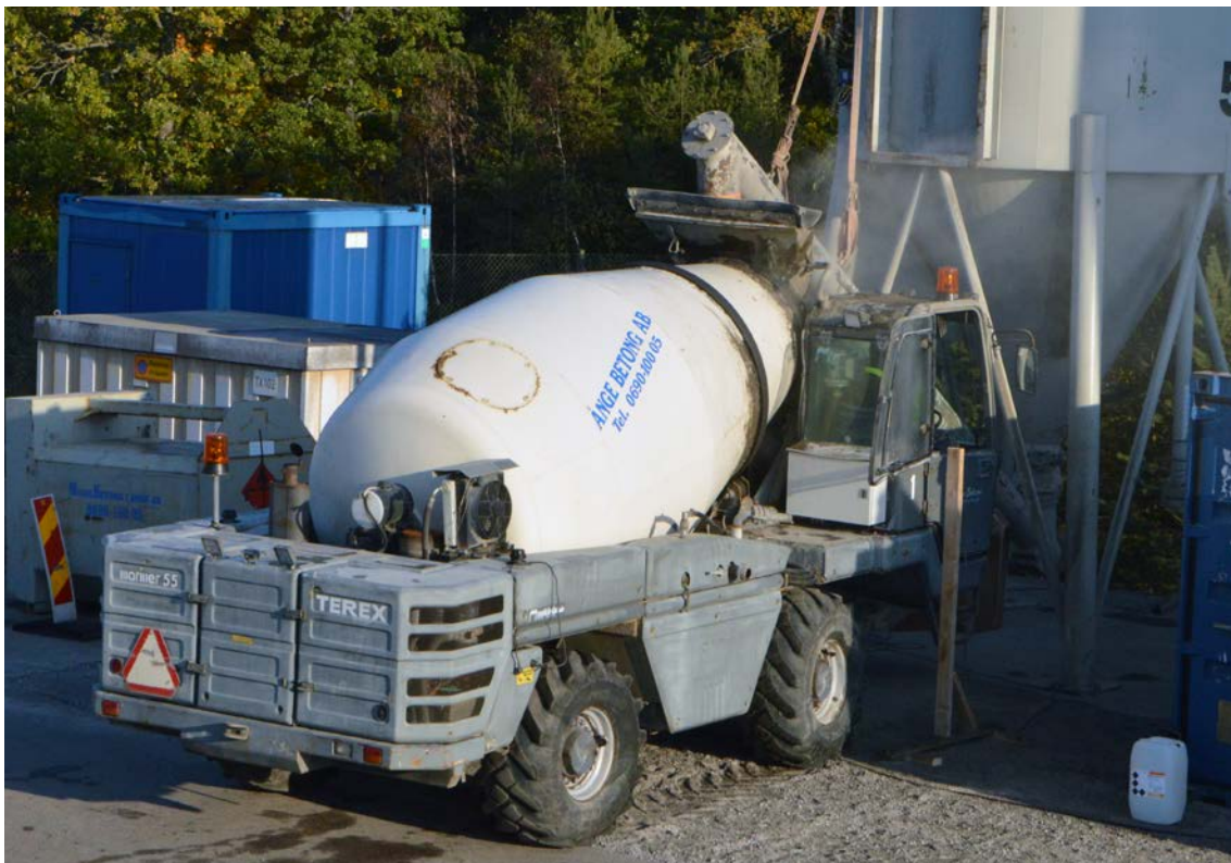
Figure 5-11. Feeding cement into the truck mixer.
