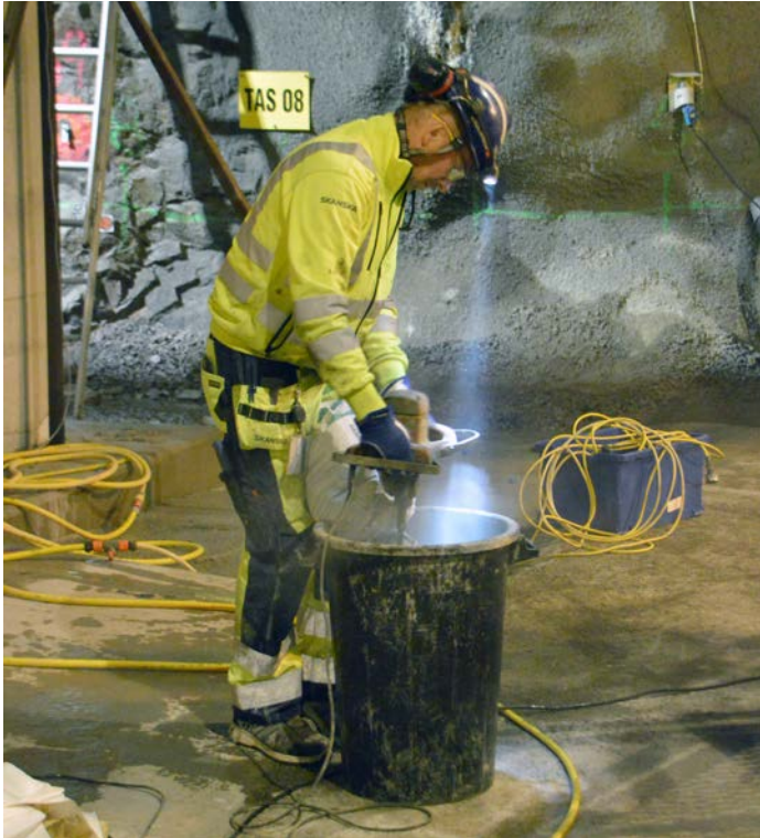
Figure 9-4. Mixing of grout.
