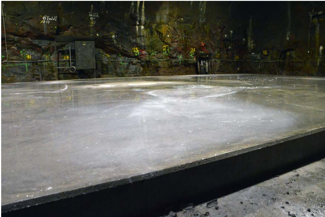
Figure 4-8. The concrete slab after grinding.
