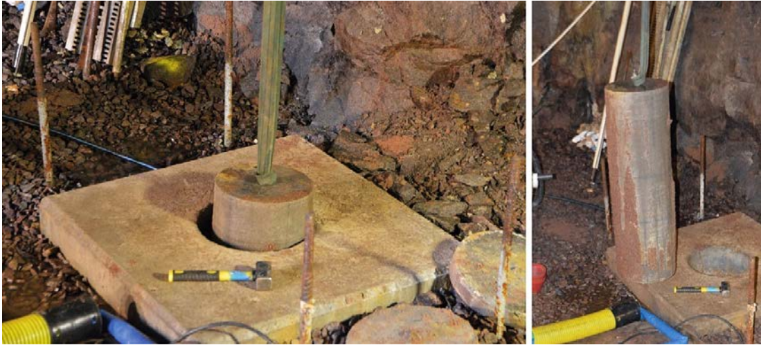
Figure 2-4. Lift of a concrete cylinder.
