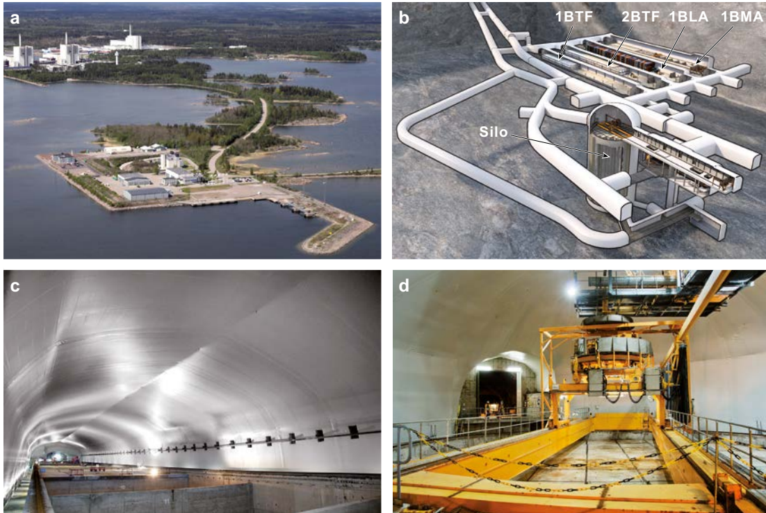
Figure 2-2. The final repository for short-lived radioactive waste, SFR, consists of two rock vaults for concrete tanks (1-2BTF), a rock vault for low-level waste (1BLA), a rock vault for intermediate-level waste (1BMA) and a silo for intermediate-level waste a) View of the surface facility, b) SFR underground, c) rock vault, d) view of silo top.
