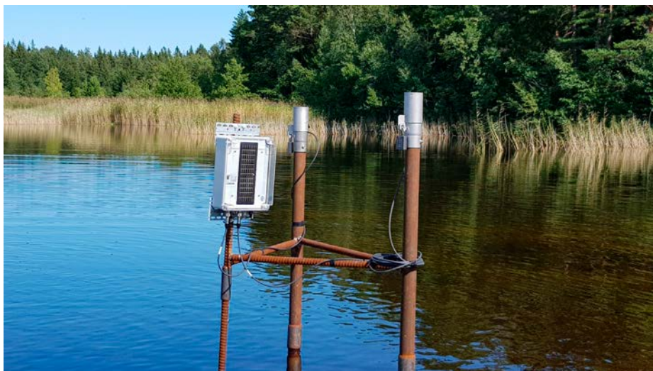
Figure 5-2. Example of installations with support rods, example from Puttan (SFM000172–173).
