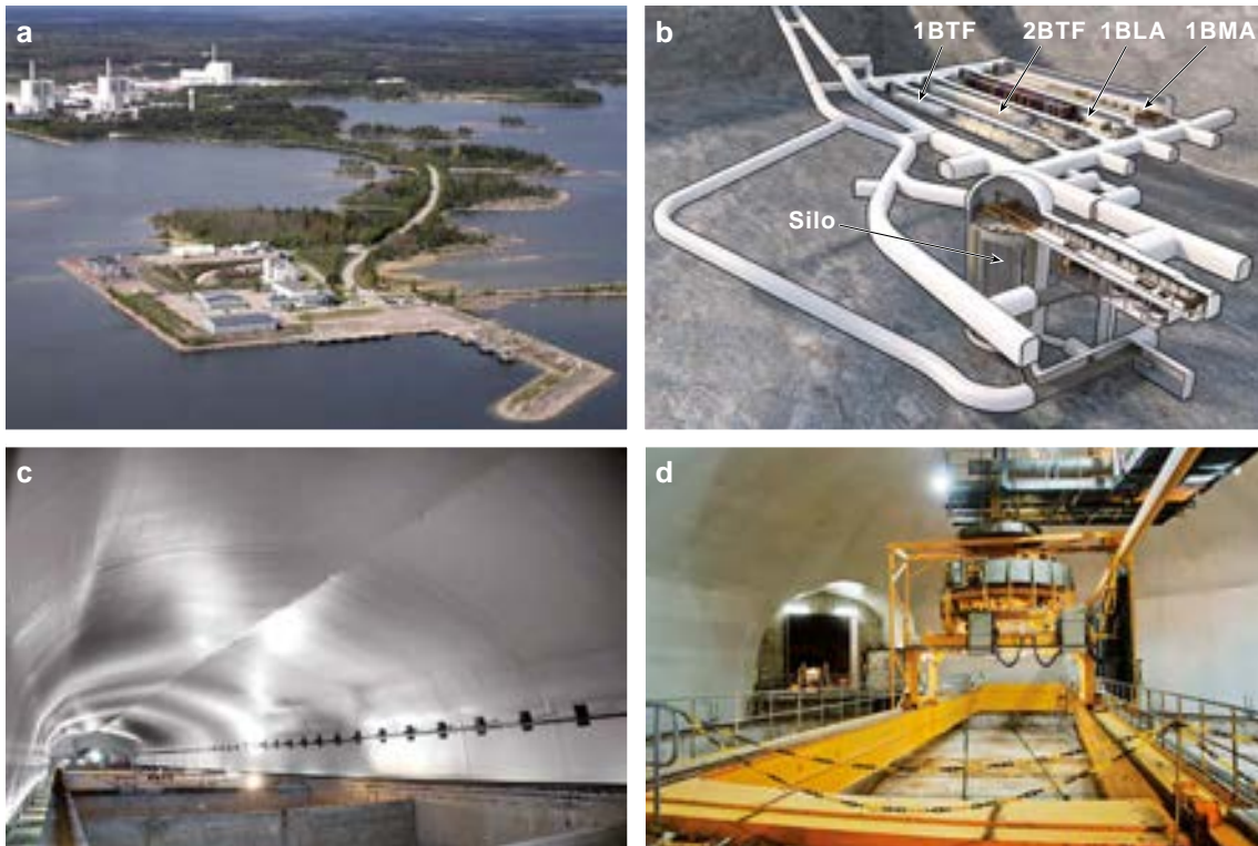
Figure 2-3. The final repository for short-lived radioactive waste, SFR, consists of two waste vaults for concrete tanks (1-2BTF), one waste vault for low-level waste (1BLA), one waste vault for intermediate-level waste (1BMA) and a silo for intermediate-level waste. a) View of the surface facility, b) SFR underground, c) Waste vault, d) View of the silo top.
