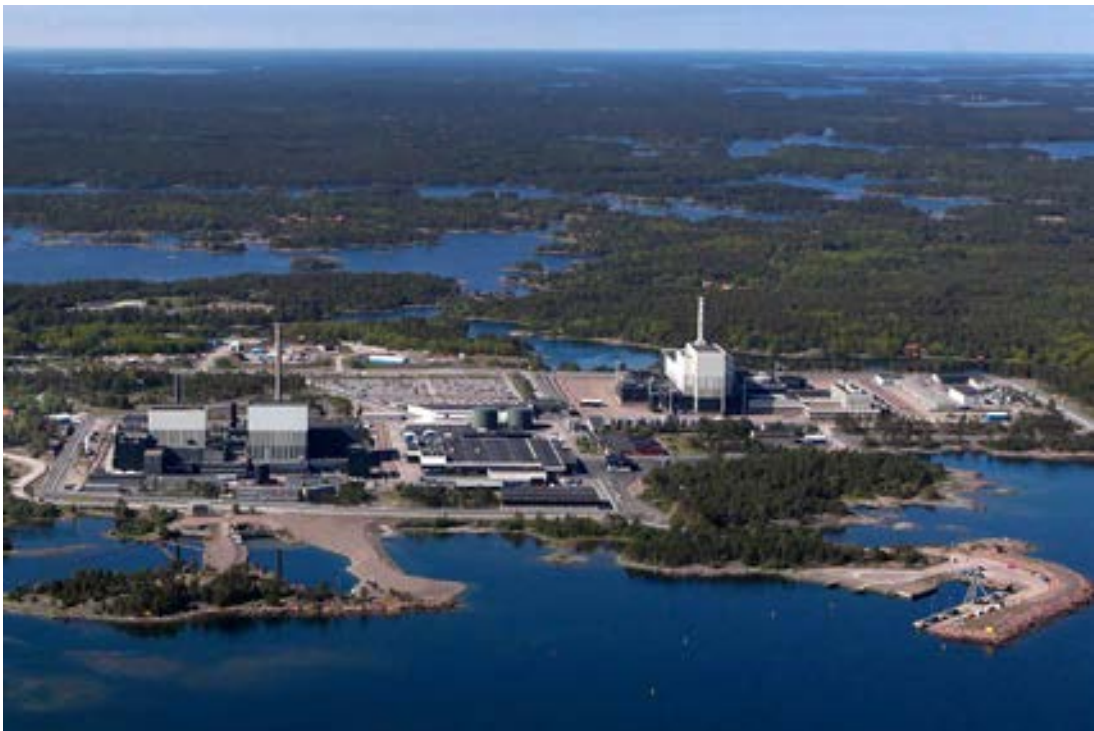
Figure 16-3. View of OKG's nuclear power plant with the three BWR reactors O1, O2 and O3 from left to right in the picture.
