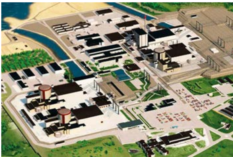
Figure 17-1. Ringhals NPP with reactors 1 and 2 to the right and reactors 3 and 4 to the left. In the centre of the site, there are office buildings and a lunch restaurant. Just above R1 in the image is the plant's waste area, which includes handling, conditioning and storage of nuclear waste.
