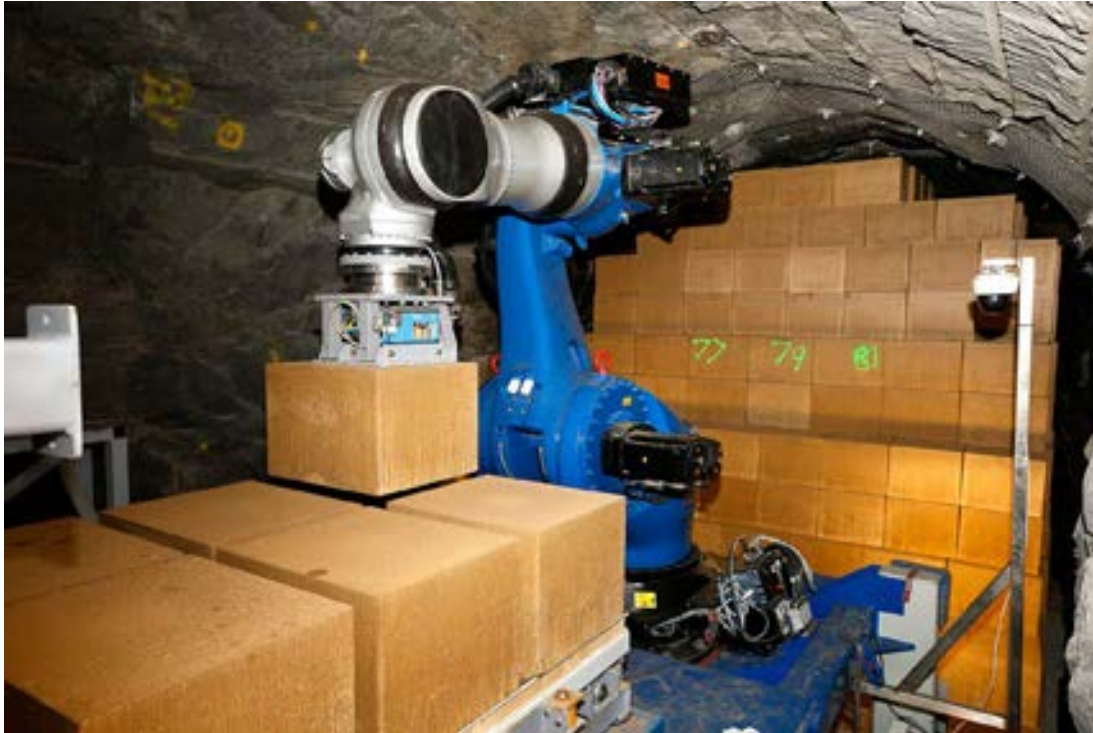
Figure 11-15. Block installation at a depth of 450 metres in the Äspö HRL.
