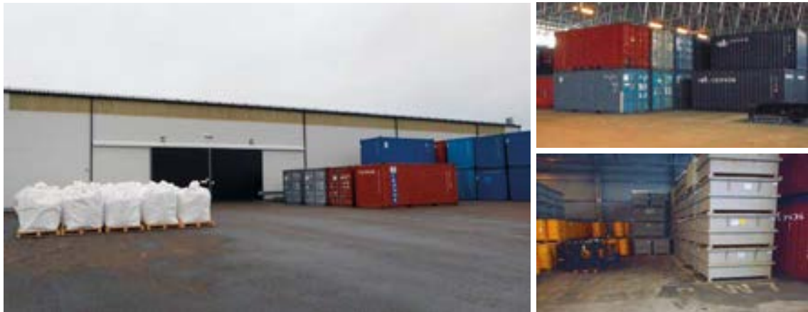
Figure 3-7. Oves Lada, temporary storage area for, among other things, very low-level waste at Ringhals nuclear power plant.
