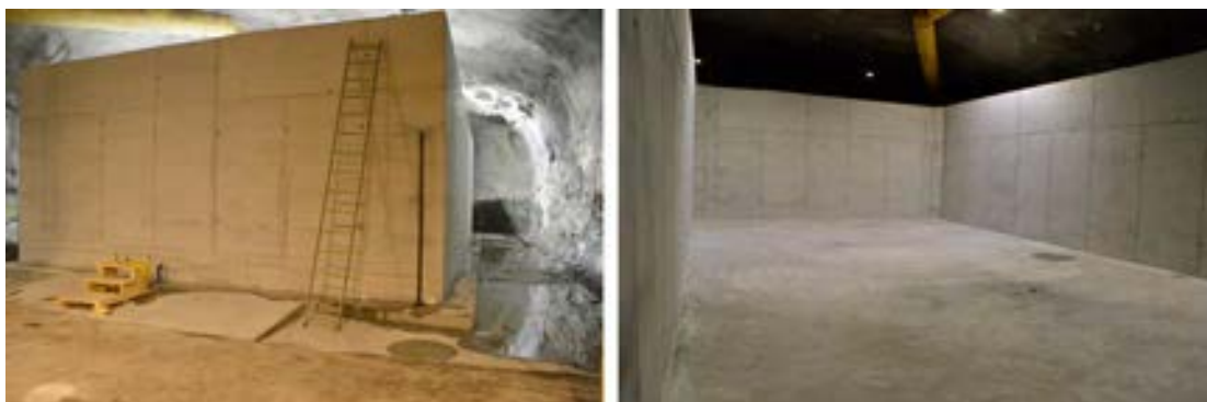
Figure 10-4. Cast caisson, outside and inside.
