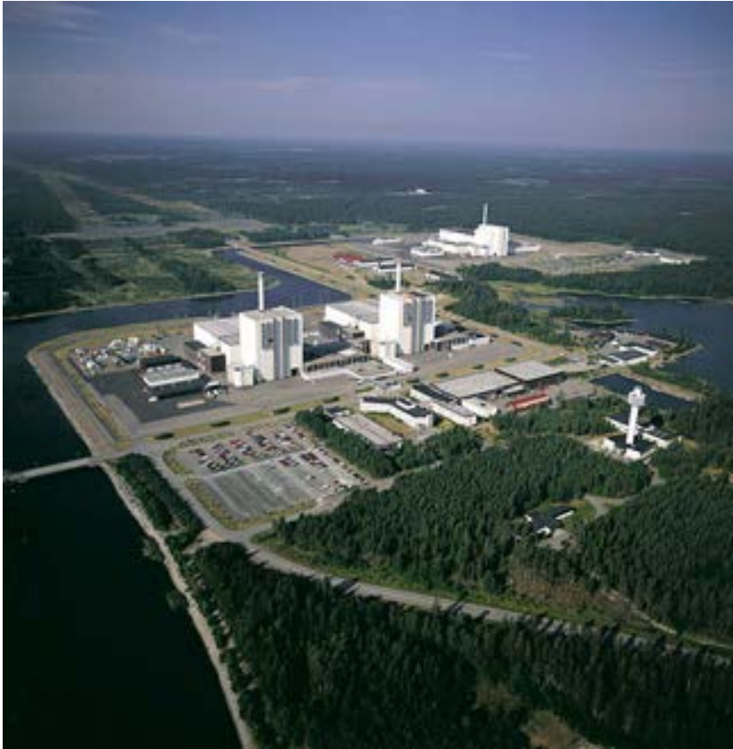
Figure 17-3. The Forsmark nuclear power plant with the three BWR reactors F1, F2 and F3, from left to right in the photo.
