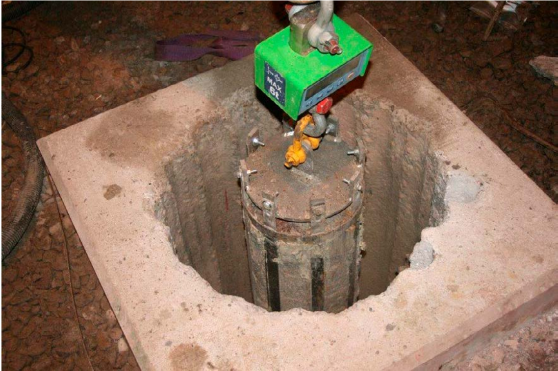
Figure 2-8. The package is lifted from the hole.
