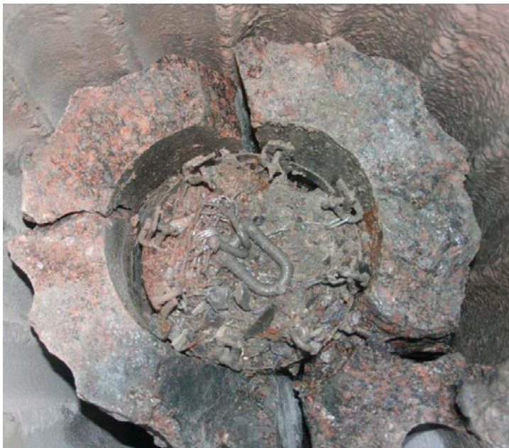
Figure 2-6. Fracturing of the exposed rock surrounding the package hampered further drilling as the drill jammed.
