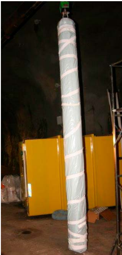
Figure 2-9. The package has been retrieved and wrapped in plastic.
