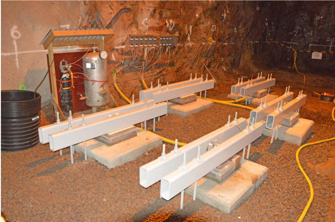
Figure 1-1. The five bentonite packages in TAS06 after completion of the installation.
