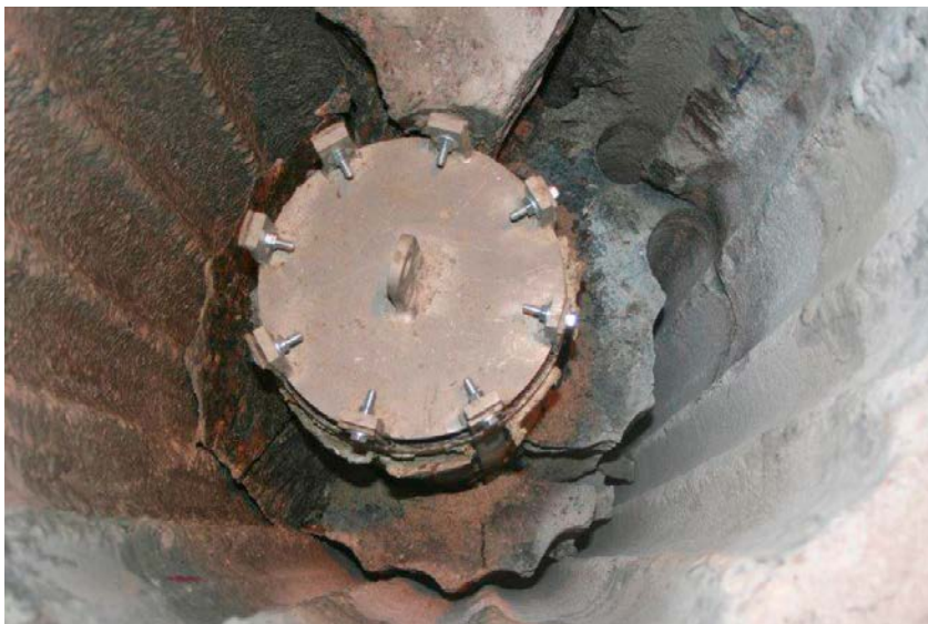
Figure 2-7. The package is sufficiently cleared to carry out a new lift attempt.
