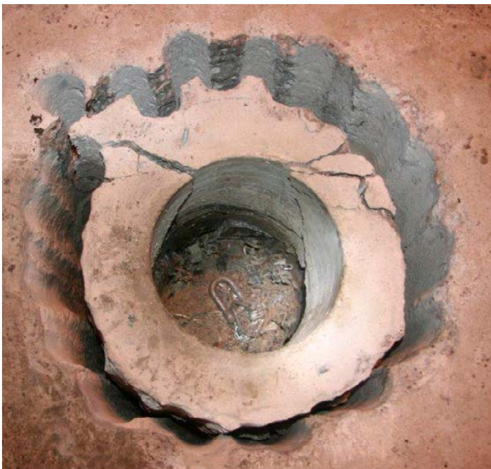
Figure 2-5. Drilling of a slit around the entire package has been completed.
