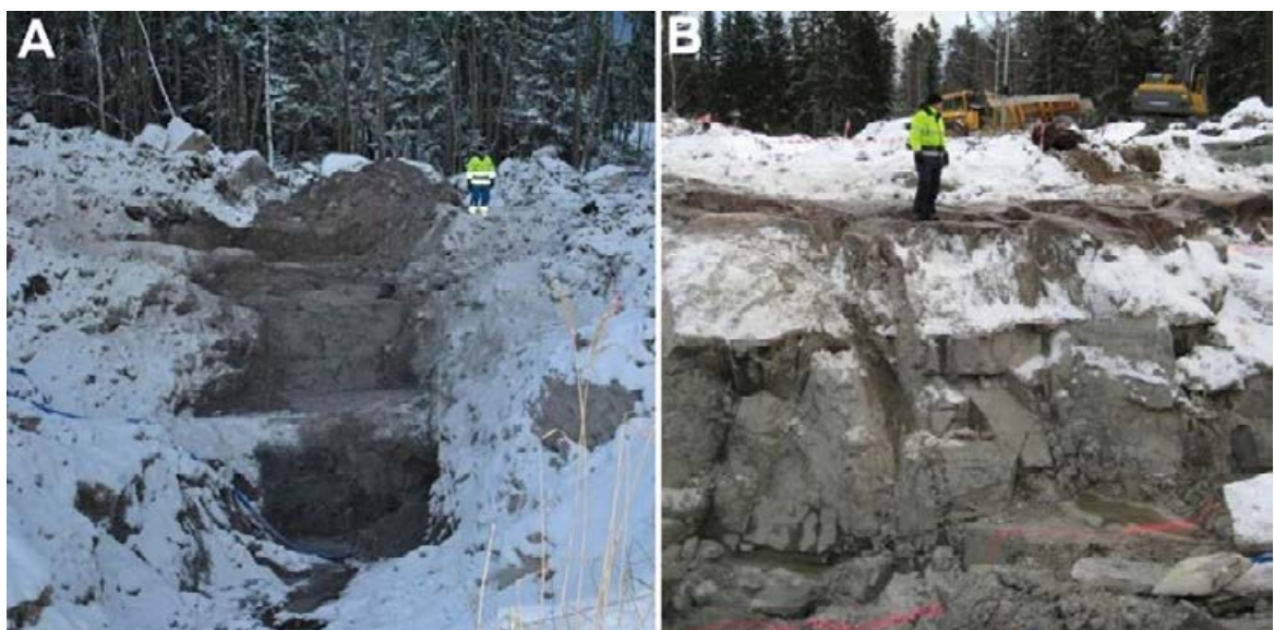
Figure 4-9. Highly varied bedrock surface in A) AFM001393 and B) AFM001394. (Photo: Lars Bergkvist, Golder Associates.)
