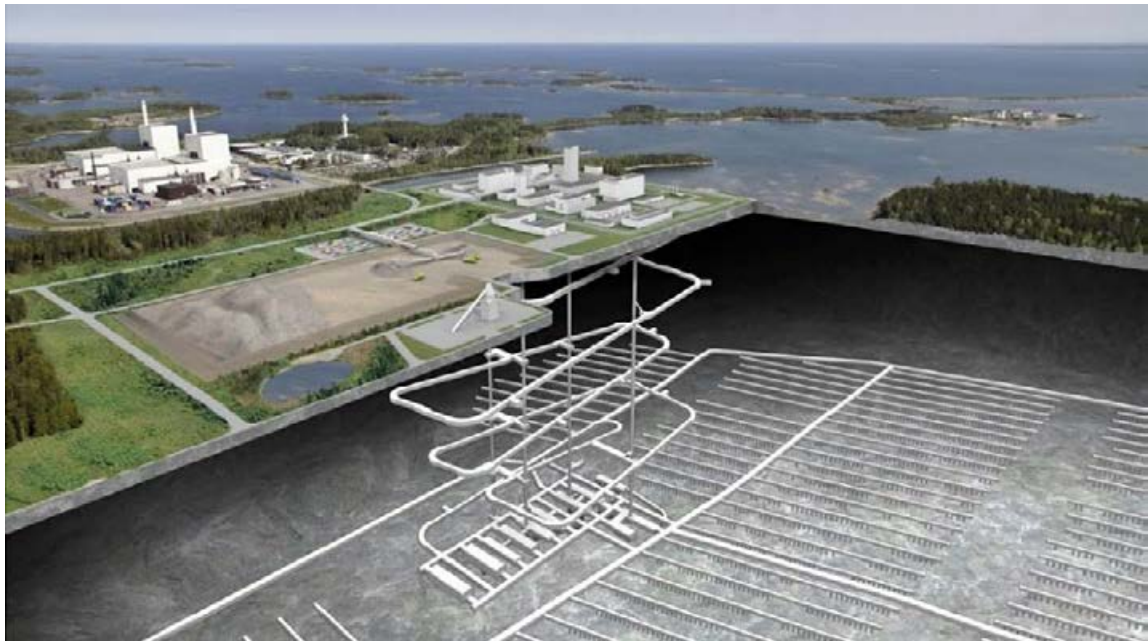
Figure 1-1. Schematic view of the access area facility part of the planned repository for spent nuclear fuel at Forsmark (Figure 2-2 in SKB 2018).
