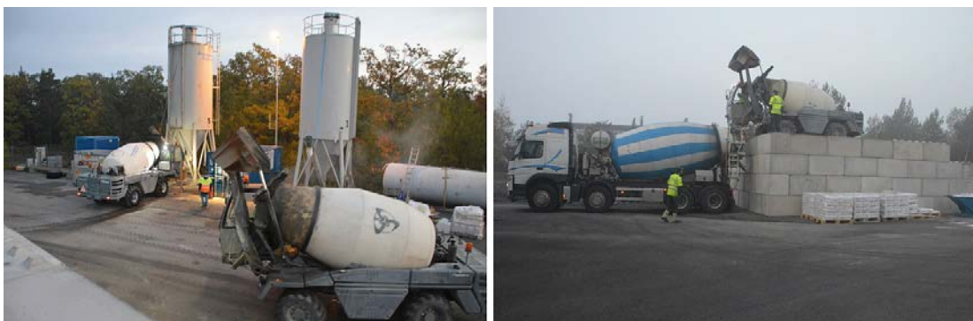
Figure 3-16. The concrete production plant and the ramp.
