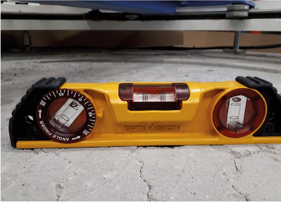
Figure 4-6. The picture shows that the milled surface for the canister is horizontal.
