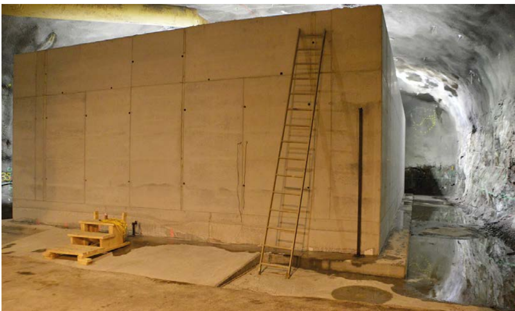
Figure 3-21. The concrete caisson after dismantling of the formwork.
