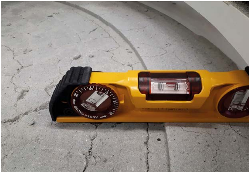
Figure 4-4. The picture shows the slope of the buffert block.
