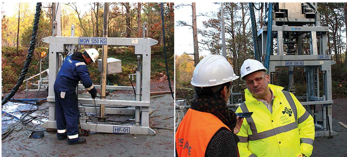
Figure 6-1. Left: installation equipment. Right: Simon Norris, senior research manager at RWM, speaking to a local newspaper.
