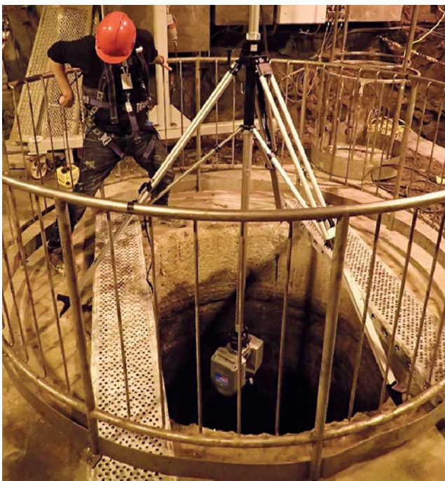
Figure 3-11. Scanning of deposition hole DO0010G01 with a Trimble TX8 Laser mounted on a rigid tripod with a downward extendable centre pole.
