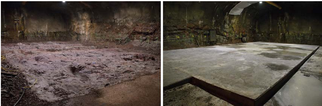
Figure 3-15. Preparations in TAS08 prior to casting of the caisson.
