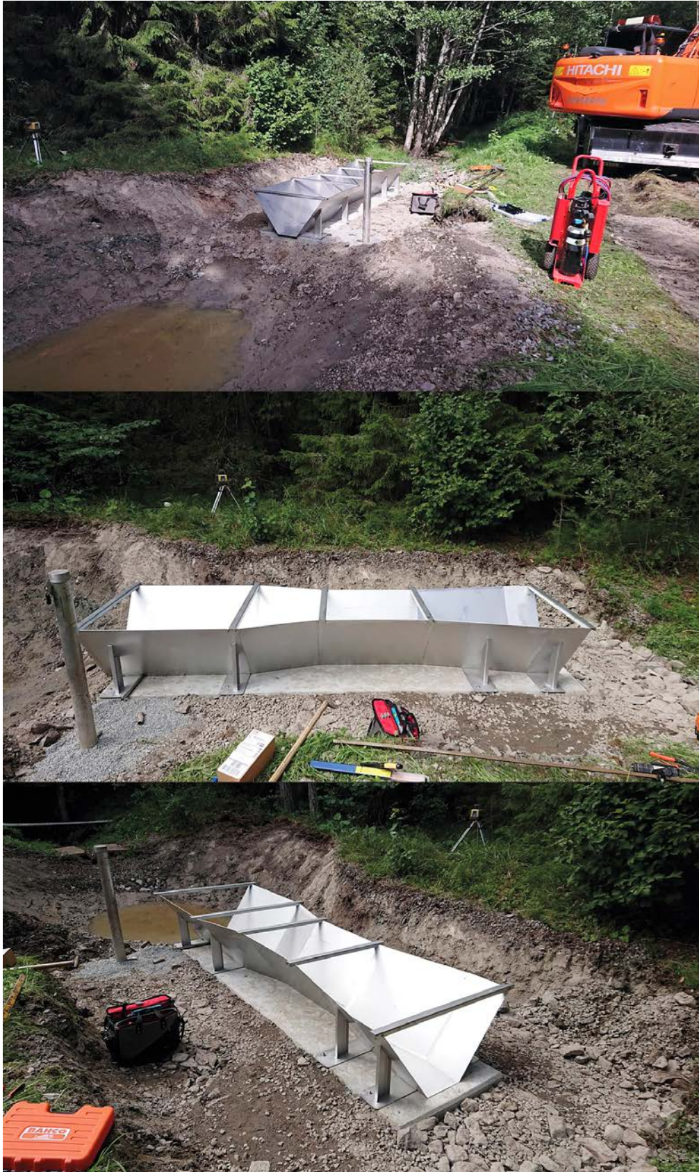
Figure 2-2. Front, side and rear views of the new flume. The front and rear views show the pool that was excavated upstream of the flume.
