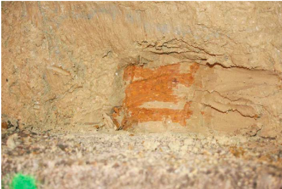
Figure 4-19. Photo showing the former pellet layer behind the LECA wall. In the photo a sample has been excavated from the pellet filling (Cebogel) and the backfill blocks (Asha) can be seen in the bottom of the hole.
