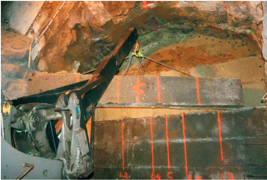
Figure 4-17. Removal of a LECA beam.
