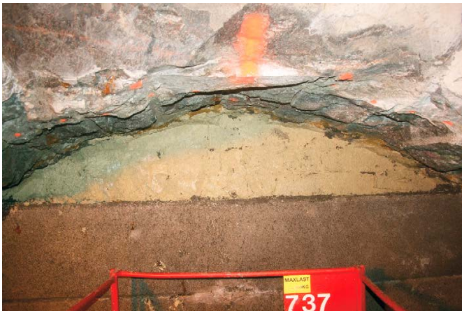
Figure 4-16. The uppermost part of the LECA wall has been removed and the backfill behind exposed.
