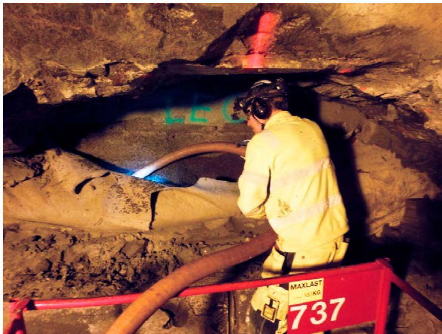
Figure 4-15. A vacuum truck was used to remove the filter material.
