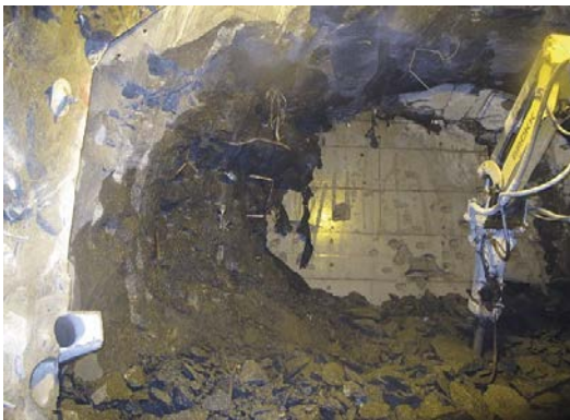
Figure 7-6. a) Concrete dome during the fourth day of demolition (2017-12-04). b) The head of the hydraulic hammer.
