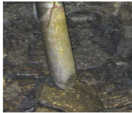
Figure 7-6. a) Concrete dome during the fourth day of demolition (2017-12-04). b) The head of the hydraulic hammer.
