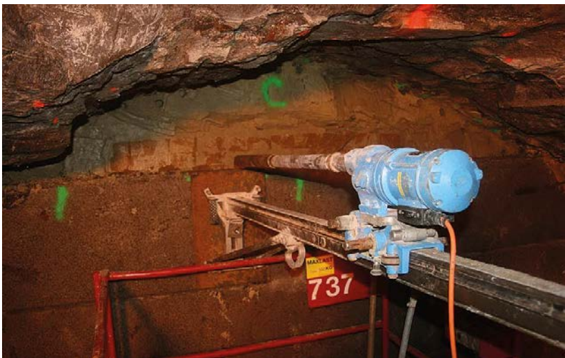
Figure 7-19. Drill used for sampling of the backfill. From Åkesson et al. (2019).
