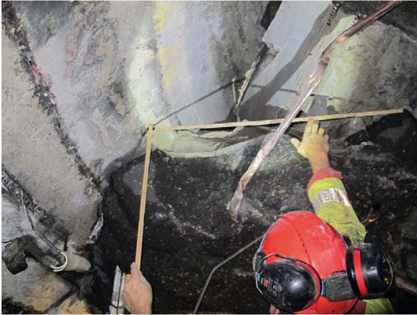
Figure 7-10. Measuring the width of the large void, about 1 m.
