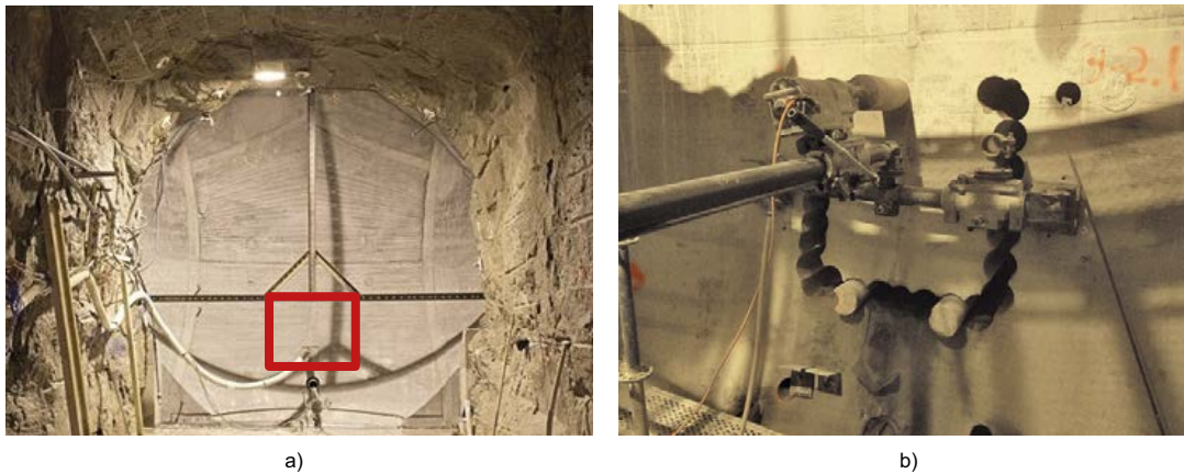
Figure 7-1. a) Location of the sample section. b) Seam drilling in progress.
