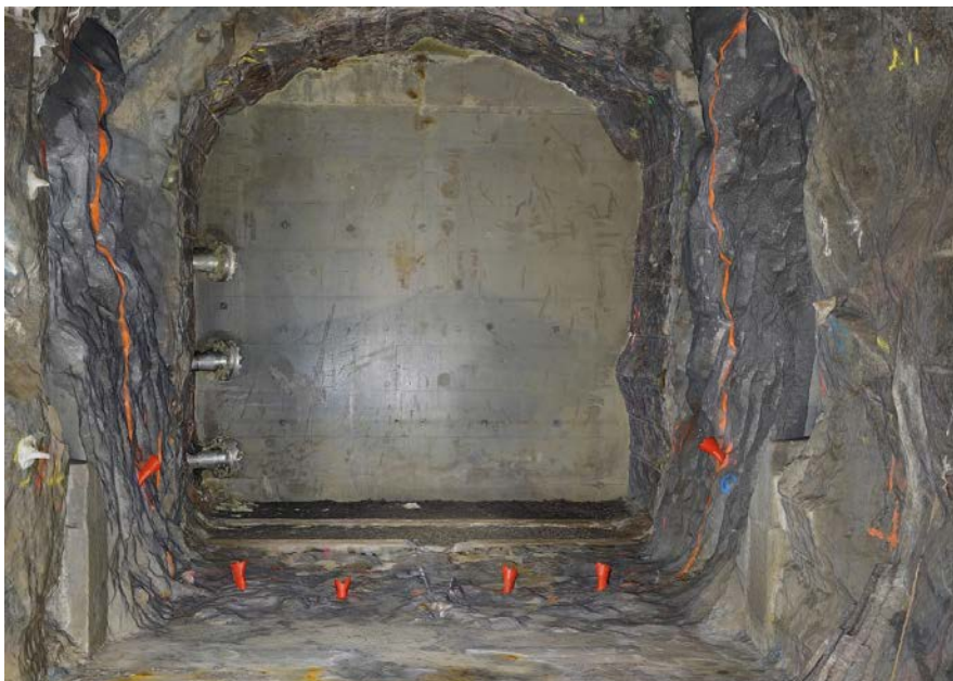
Figure 7-21. Photo of the tunnel after demolition of the plug.
