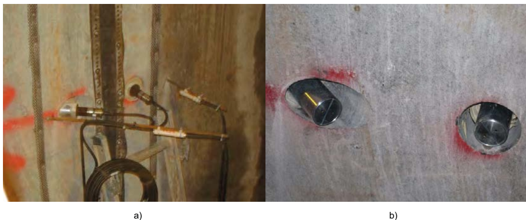
Figure 2-19. a) Illustration of two joint meters and two strain gauges mounted on reinforcement bars and b) The sockets used for the joint meters (Malm 2015a).
