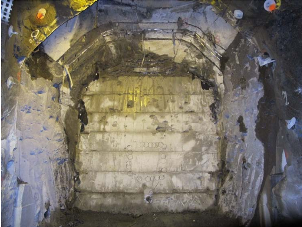
Figure 7-8. The concrete dome after the 14th day of demolition.
