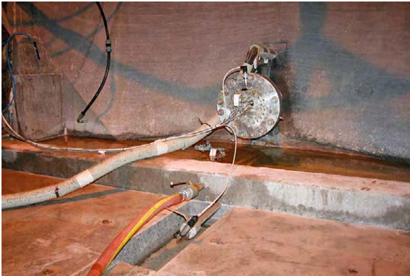
Figure 2-11. A photo of the downstream leakage weir.
