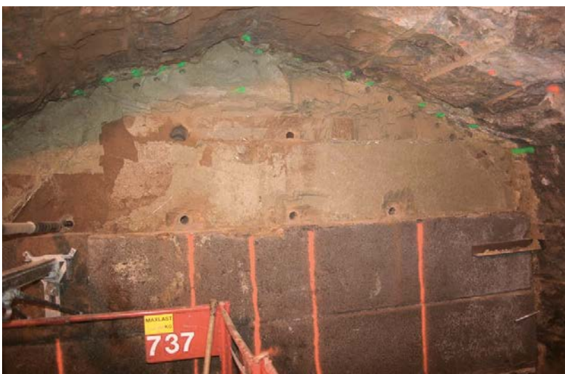
Figure 7-20. The upper part of the backfill after two LECA beams has been removed a number of samples have been taken. From Åkesson et al. (2019).
