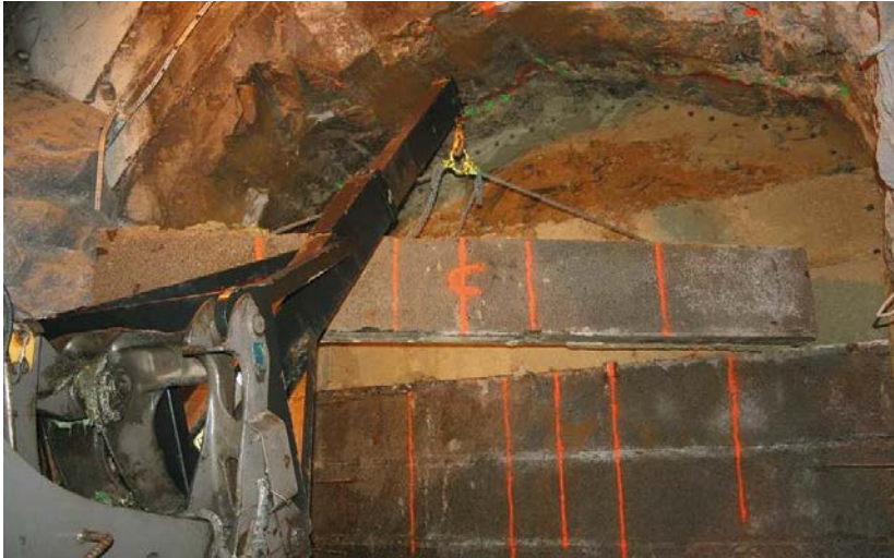
Figure 7-18. Removal of a LECA beam.
