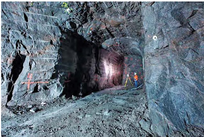
Figure 2-3. Photo of the finished experiment tunnel (Grahm et al. 2015).
