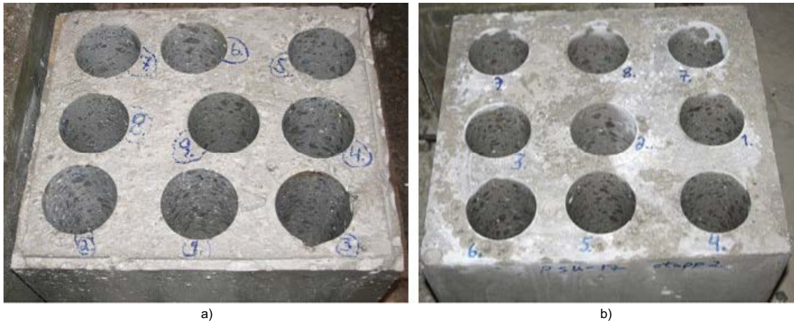
Figure 1-1. Small cube cast from concrete from truck #7 in Section 1 (a) after drilling of cores for further testing (ETAPP1), and from truck #4 in Section 2 (ETAPP2) (b).
