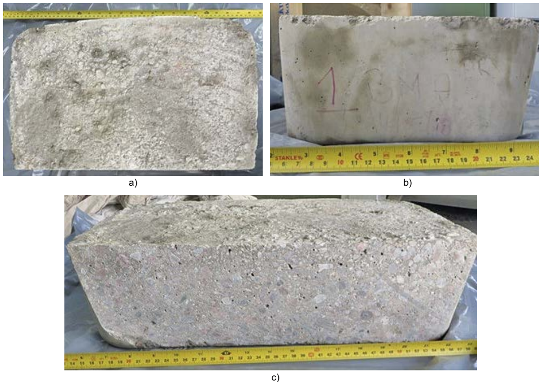
Figure 2-4. BMA concrete sample without packaging. Top (a) and lateral (b) view; appearance of the section of the sample BMA.
