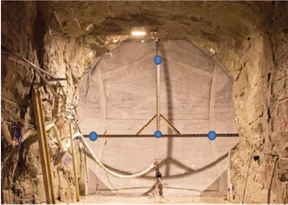
Figure 3-11. Illustration of additional LVDT sensors installed prior to the leakage test.
